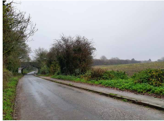
View looking north east towards the setting along St Mary's Well Bay Road illustrating enclosing nature of disused railway embankment
