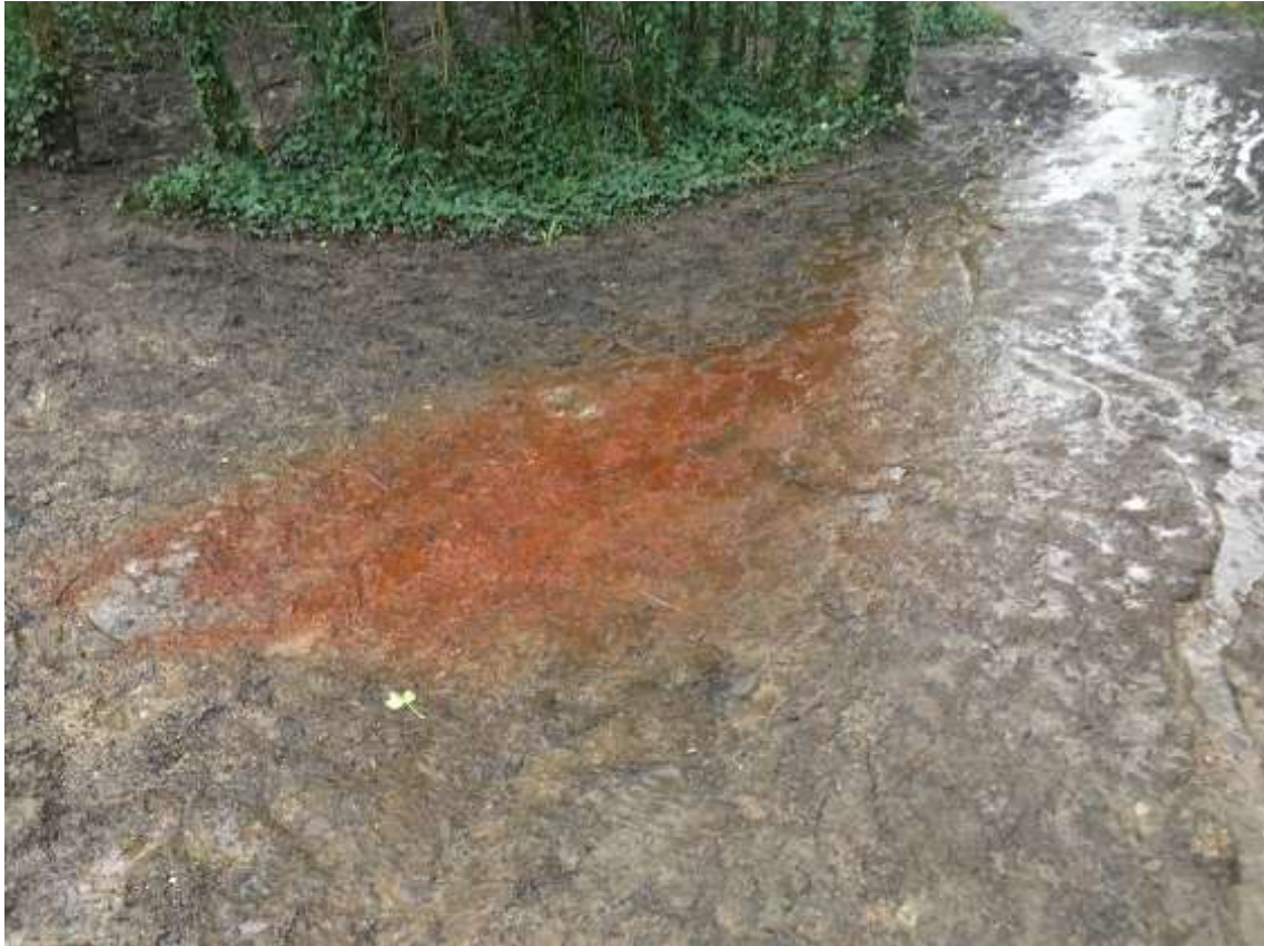
The ground Leachate level is rising and now exiting in the middle of the pedestrian walkway
