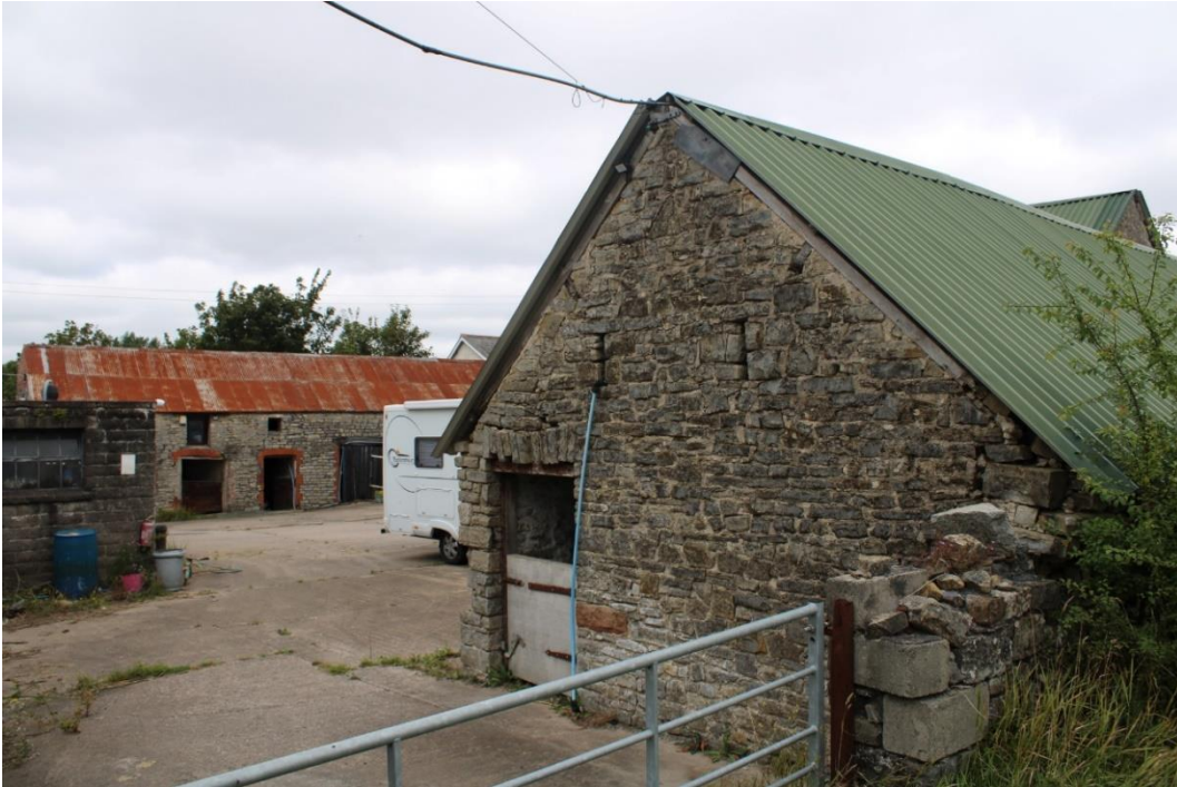
Photo 19: Looking north across the western gable end of the southern building of the courtyard, with the 17 th century farmhouse behind across the courtyard
