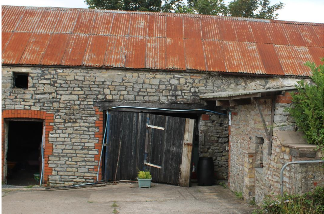
Photo 5: Looking north at the inserted double doored cart entrance to the earliest phase of the 17 th century farmhouse
