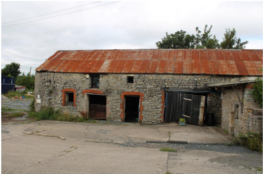
Photo 1: Overview of southern façade of Lower Cosmeston Farmhouse
