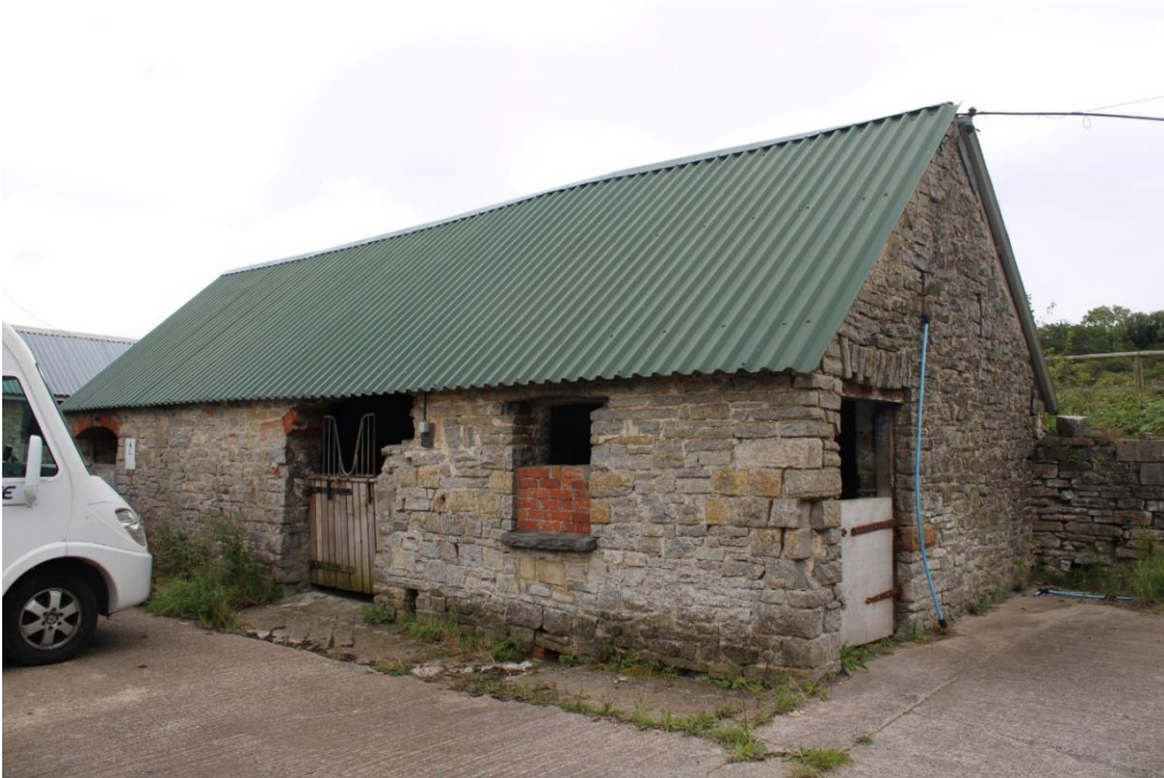
Photo 18: Looking southeast across the southern building of the courtyard
