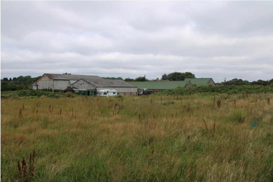
Photo 23: Looking northeast across Lower Cosmeston Farm showing modern sheds to right and metal roofs of courtyard buildings to centre from field where school is proposed
