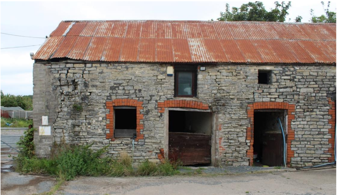
Photo 4: Southwestern side of 17 th century farmhouse showing central and western wide door, with flanking window and windows above doorways and with rebuilt western gable end
