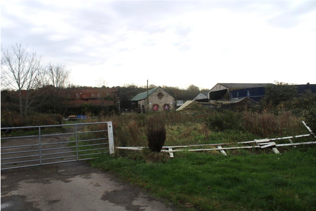
Photo 21: Looking south across Lower Cosmeston Farm showing the western stables building with the 17 th century farmhouse to left and modern metal sheds to the right (24.11.2020)
