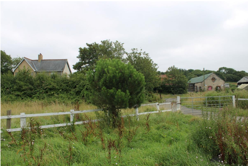
Photo 22: Looking south across Lower Cosmeston Farm showing the western stables building to the right with the 17 th century farmhouse centre and modern farm,house to left
