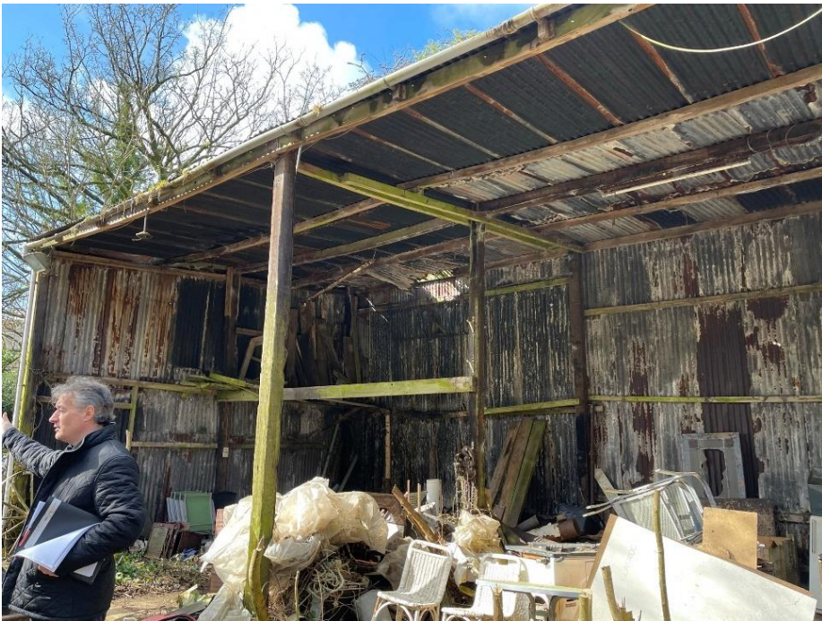
Large dilapidated corrugated barn to be removed and replaced with two smaller lodges
