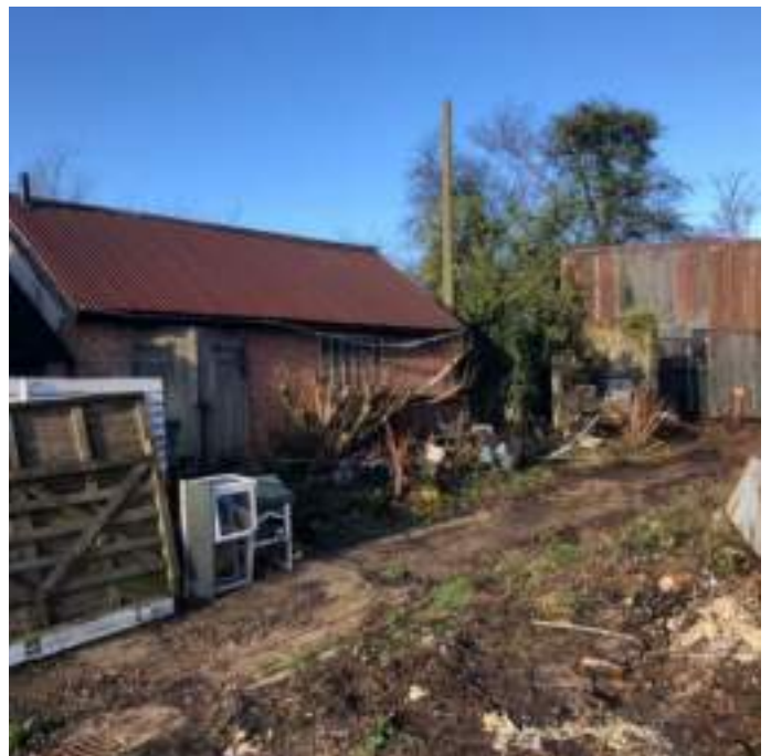
Image of both buildings to be converted together
