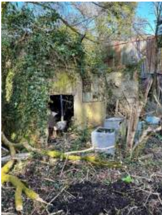
Grey Brick Building (to be converted)
