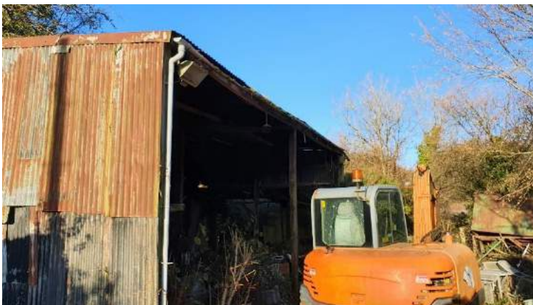
Figure 3-16 Looking north showing the existing buildings
