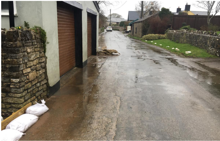
Figure 9-5: Existing Drainage, @photograph from AECOM site visit
