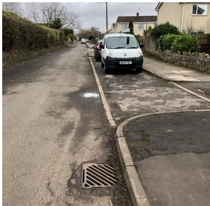
Figure 9-3: Existing West Road Drainage @photograph from AECOM site visit
