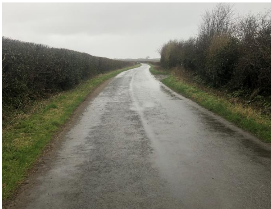
Figure 9-1: Existing Sigingstone Lane, @photo from AECOM site visit
