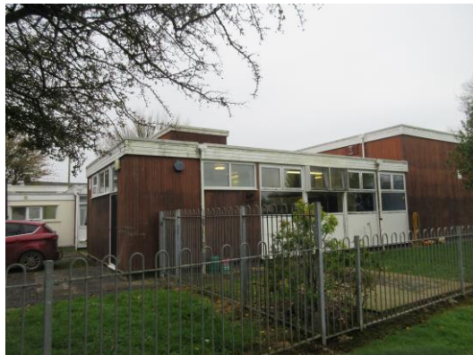
Plate 2: Main School Building
