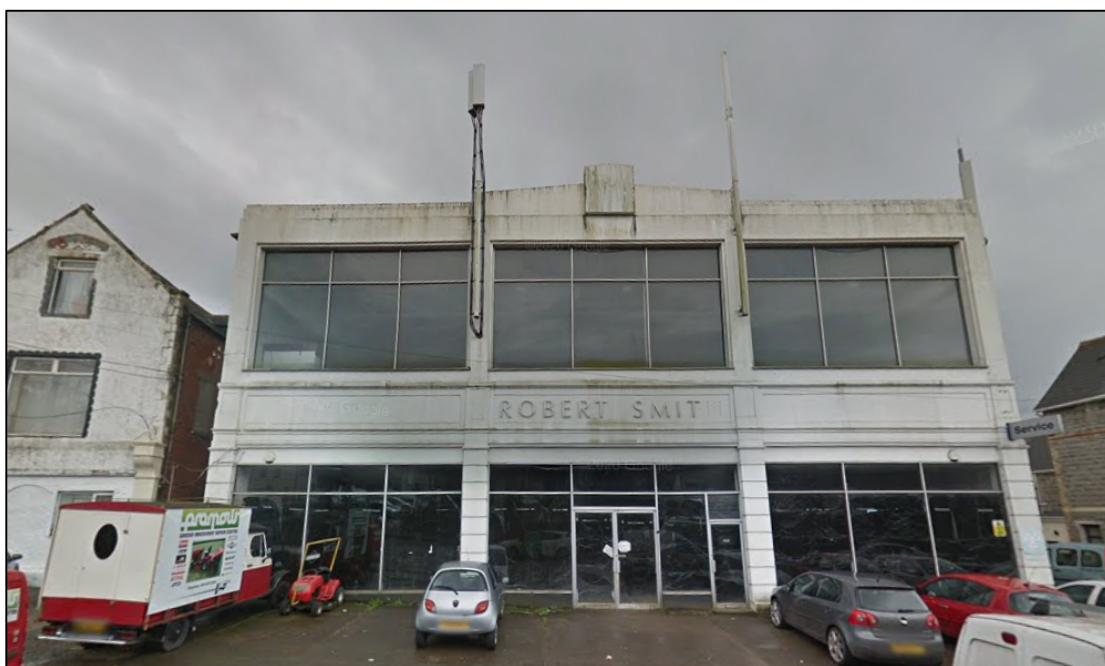
Figure 1: View of the Robert Smith building before redevelopment from Windsor Road
