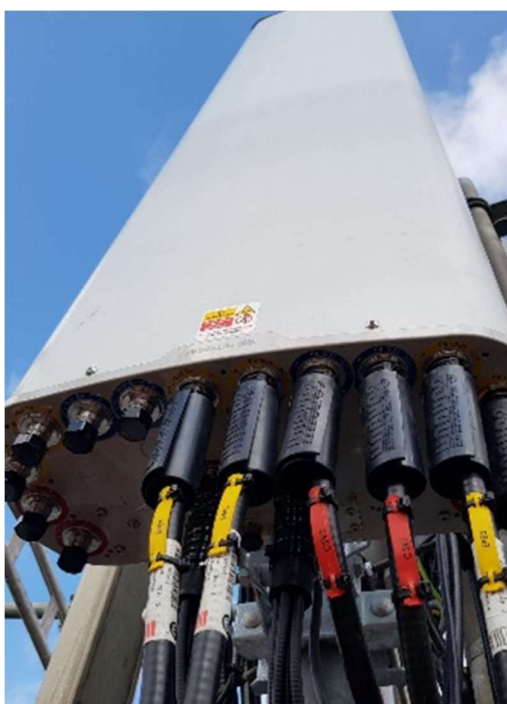
Source: Cellnex Trowell Services – 5G antenna and feeders
