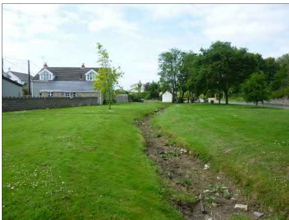
Figure 3-3: Channel Cross Section Through the Village Green at Llanmaes (Manning's Roughness Coefficient of 0.041)
