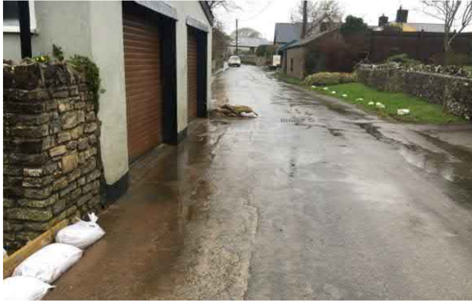
Figure 9-5: Existing Drainage, @photograph from AECOM site visit
