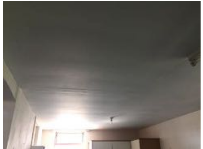
internal view of flat roof area
