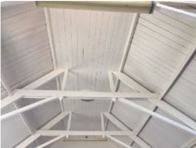
Internal view of roof
