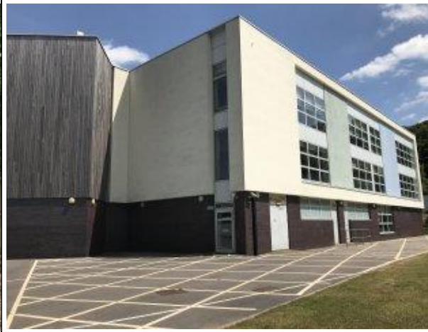
Photograph 26: Building 12 (Block A).
