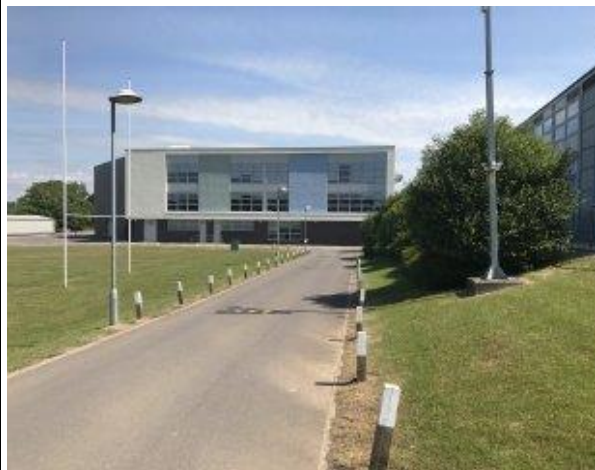
Photograph 27: Building 12 (Block A).
