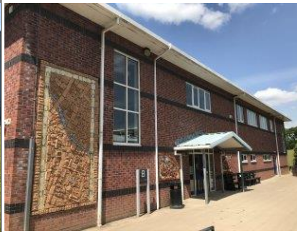
Photograph 28: Building 14 (Block B).
