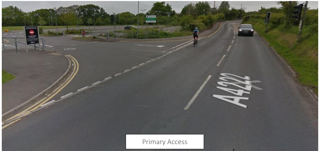
Figure 2-2: Existing Site Accesses – Aberthin Road
