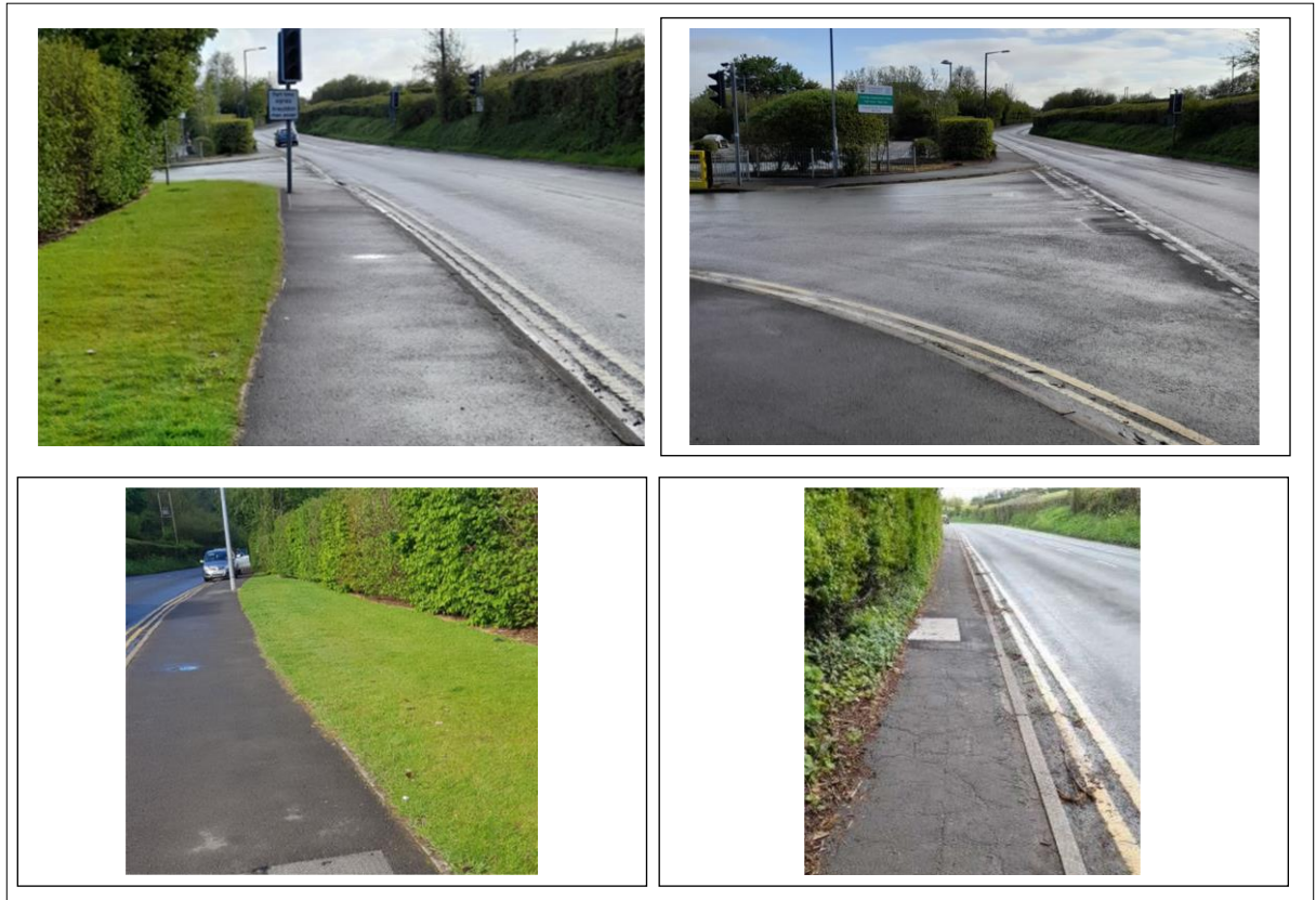
Figure 3-1: Existing Footways along Aberthin Road
