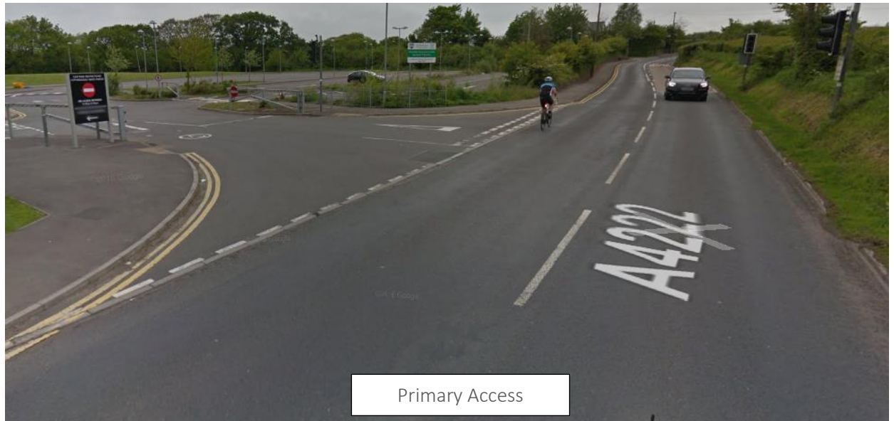
Figure 2-2: Existing Site Accesses – Aberthin Road
