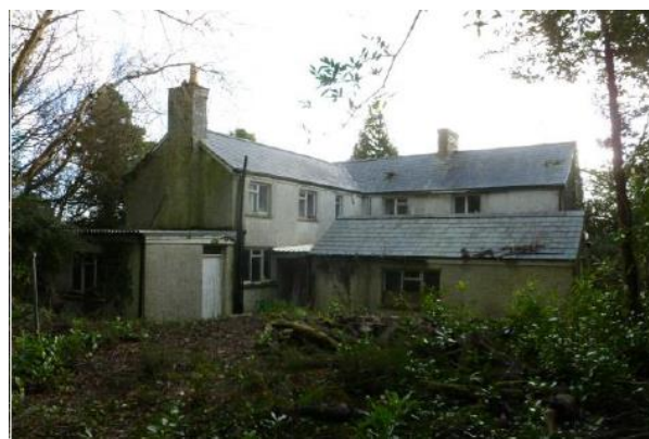
Rear Elevation of Bolston House
