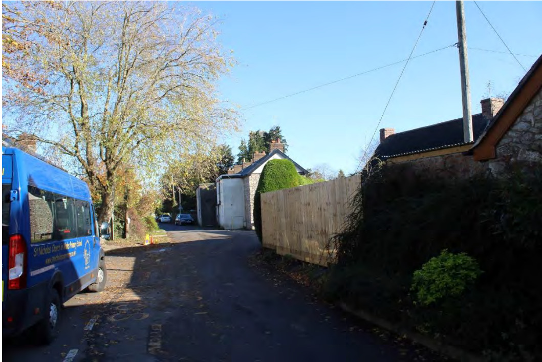
Photo 3: View east along School Lane in front of school
