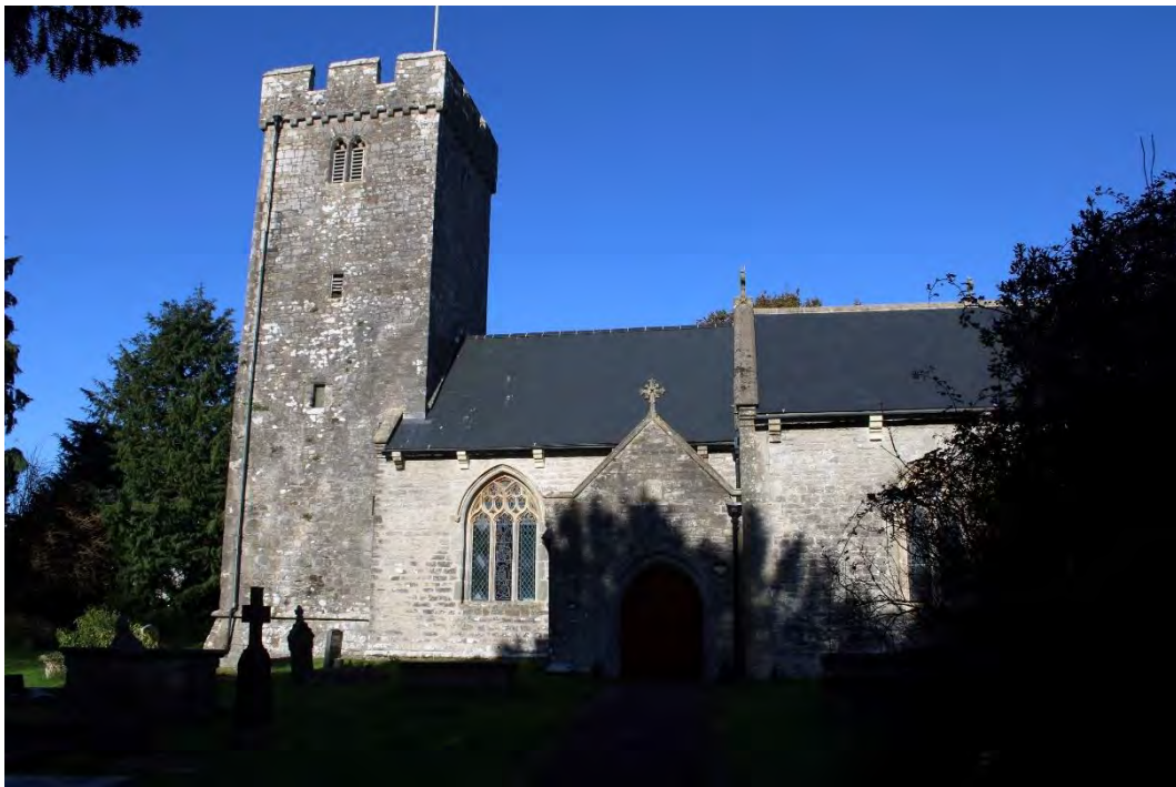
Photo 18: View north of Parish Church of St Nicholas showing west tower
