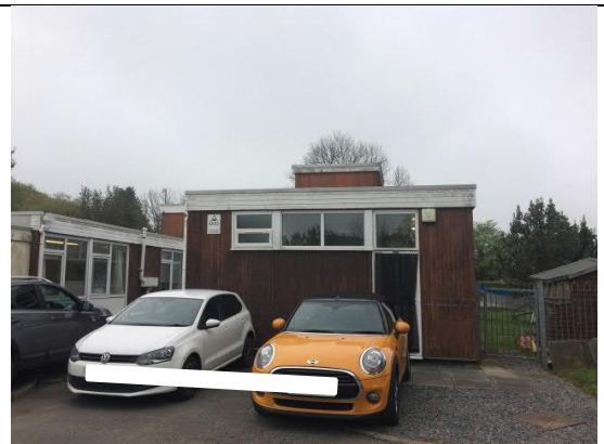
Photograph : Building 4 – showing elevated central roof section
