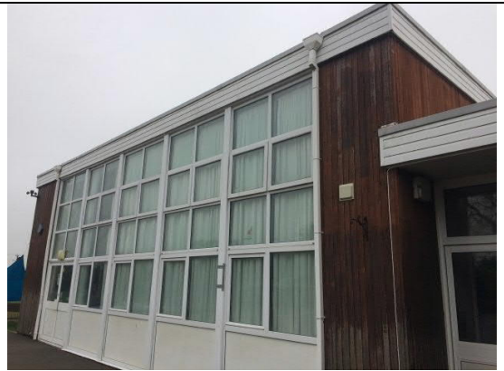
Photograph : Building 4 – School Hall
