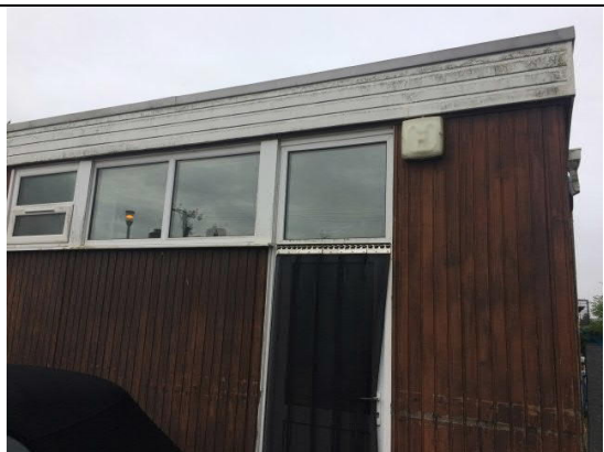
Photograph : Building 4 ,East Face
