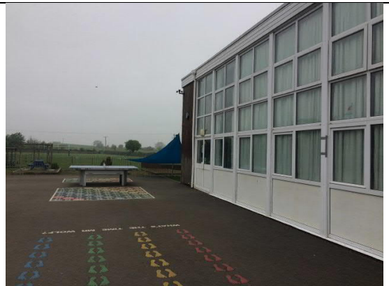
Photograph : Building 4 – School Hall
