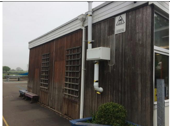
Photograph : Building 1 – west face
