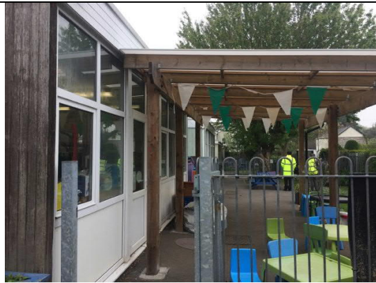
Photograph : Building 1, south face
