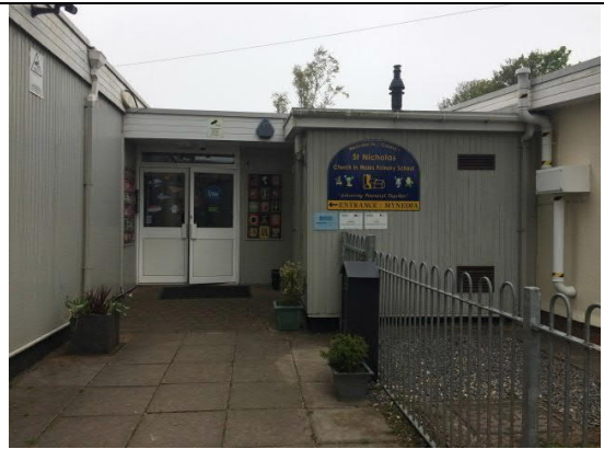
Photograph : Building 1, south face. School entrance.
