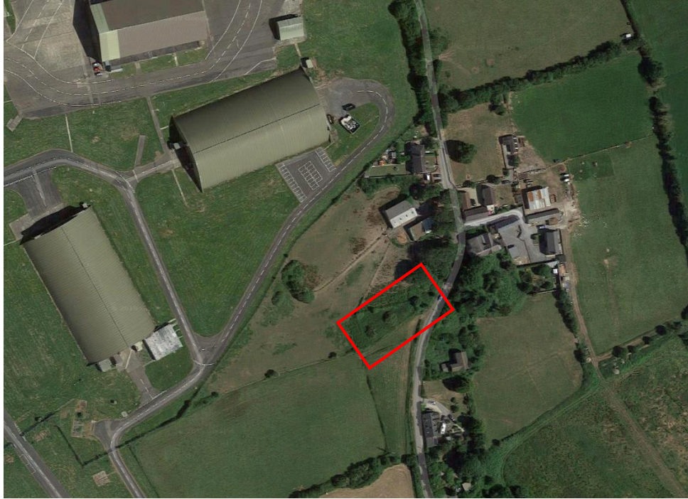
Figure 6: The images below shows where the land level rises which obscures views onto the development site. (Source: Google Maps 2019).
