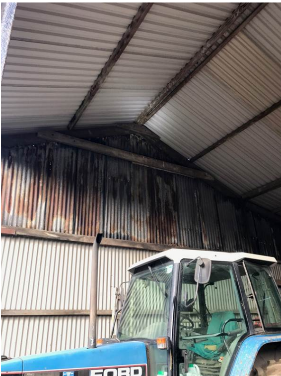
Figure 2 Internal structure of Barn D
