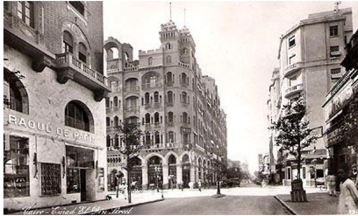
Figure 21 - The St David Building, Cairo (1910)
