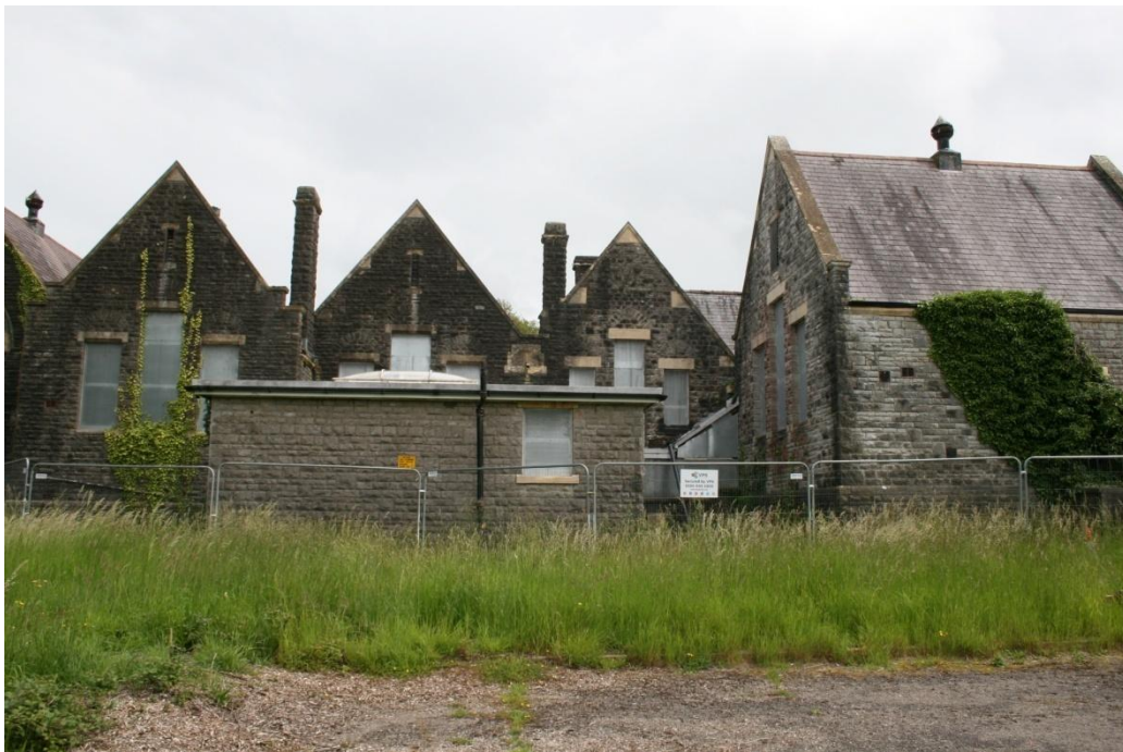
Figure 17 - rear elevation showing survival of chimneys and ridge-vents
