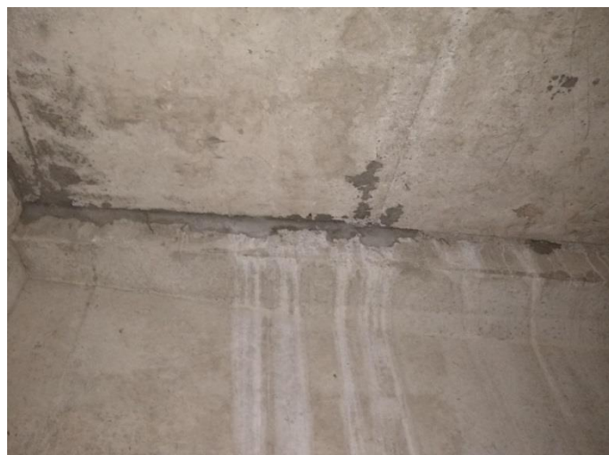
Plate 2 – Repair works and blocking of gaps
