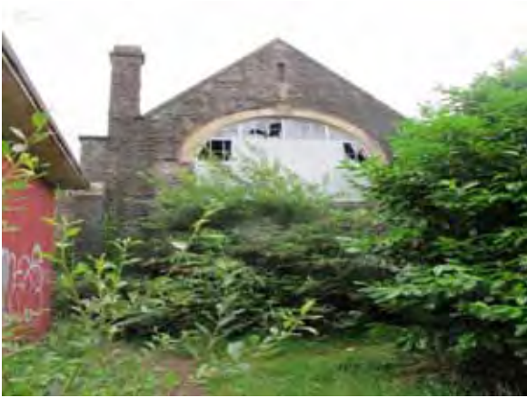
End gable on north-west aspect
