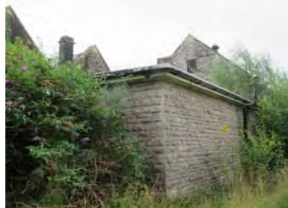
Flat roof room to rear of main school building
