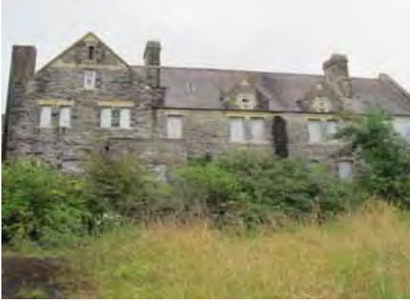
Main school building, north-west aspect
