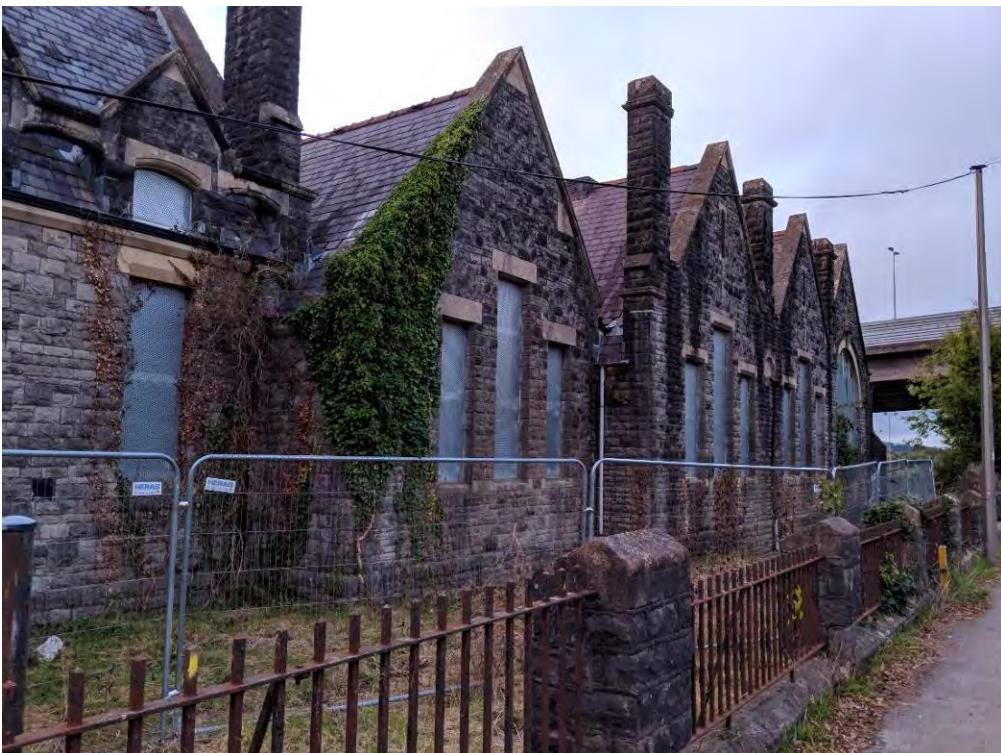
Image EDP 8: South-east facing elevations of the north-east end of the school building.
