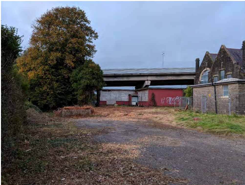
Image EDP 14: Image showing the two remaining 1950s buildings and the stone wall remnant of the older outbuilding.
