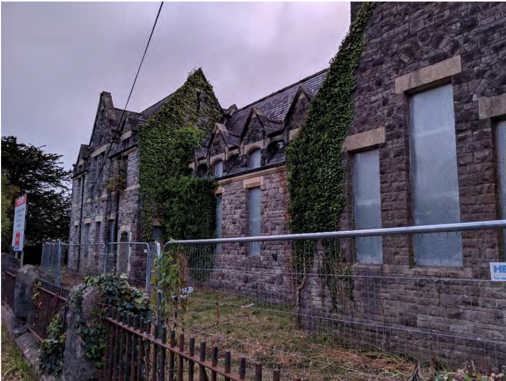
Image EDP 7: South-east facing elevations of the south-west end of the school building.
