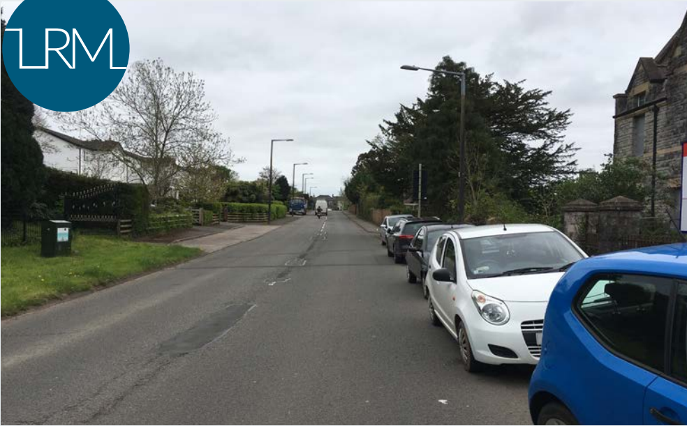
Figure 16 - View southwards along Aberthin Road
