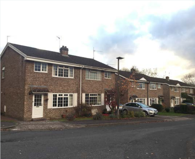
Figure 20 - Dwellings on Millfield Drive
