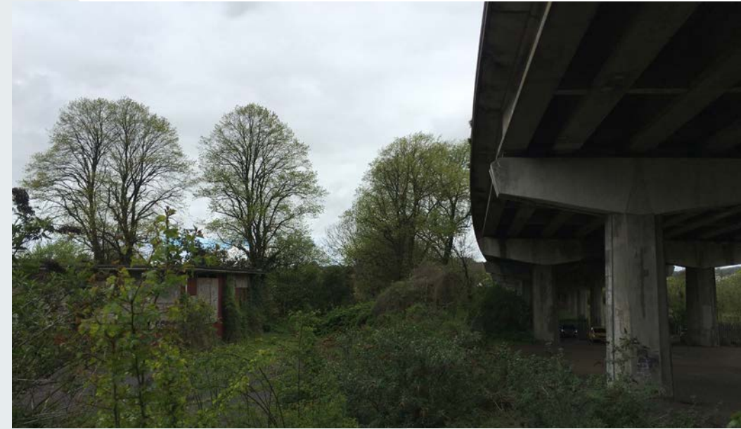
Figure 17 - Northern part of site alongside flyover, demountable structure visible to left-hand side
