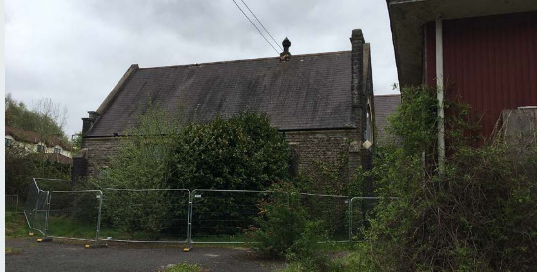
Figure 10 - View of side (northern) elevation with demountable structure visible on right-hand side
