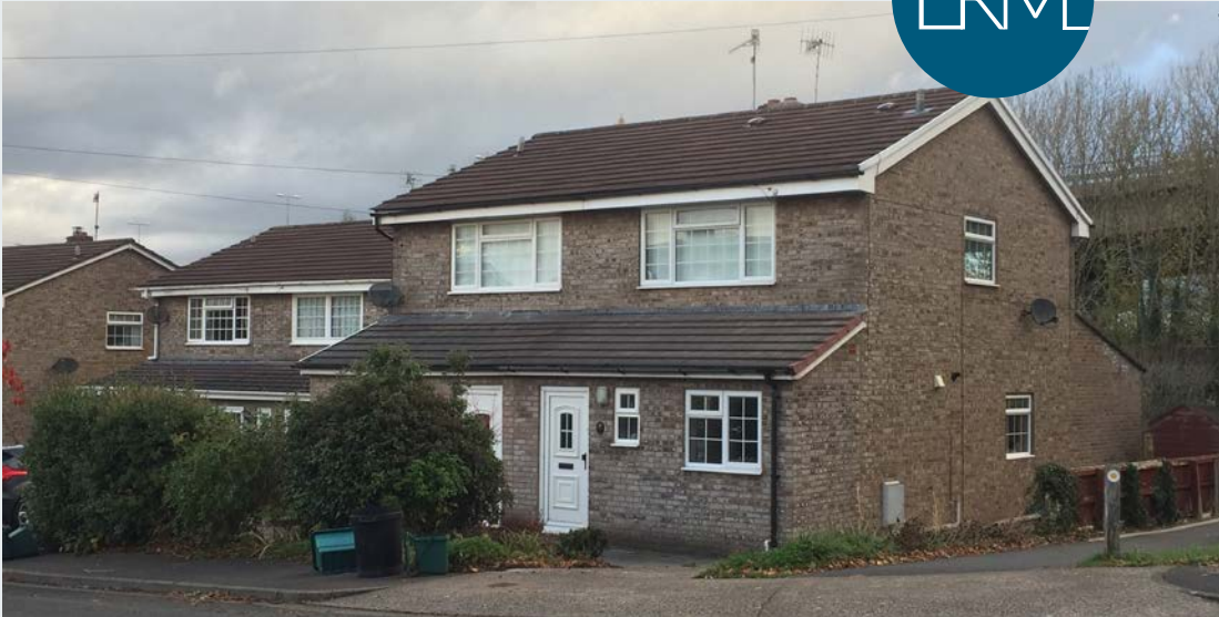
Figure 21 - Dwellings on Millfield Drive, flyover visible to rear
