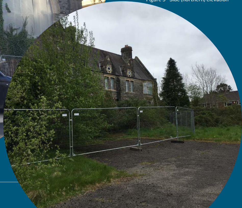
Figure 5 - Side (northern) elevation
