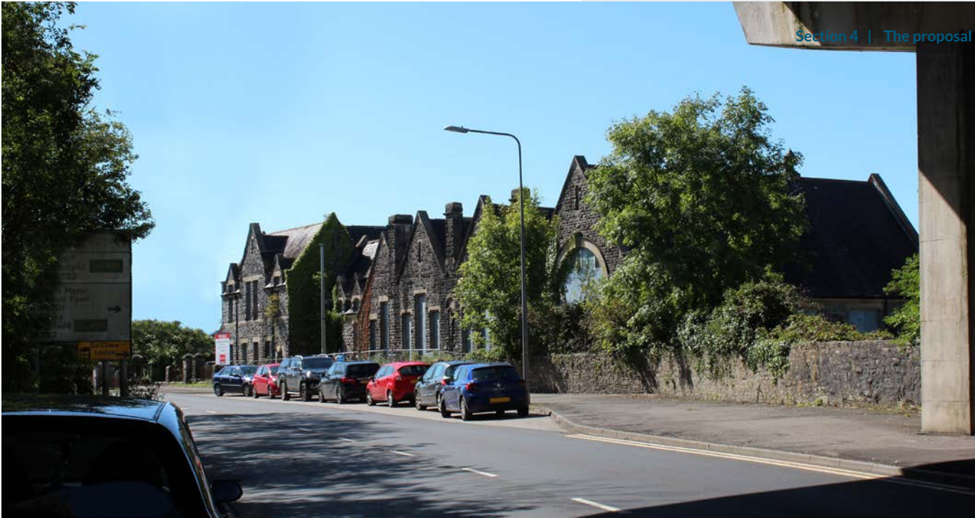
Figure 46 - Current view from north along Aberthin Road
