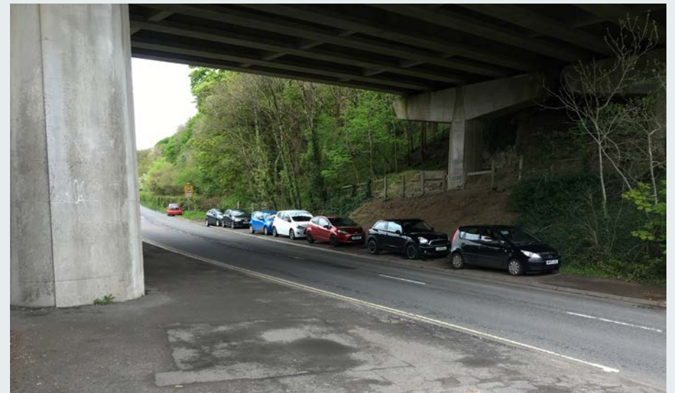
Figure 31 - View underneath flyover
