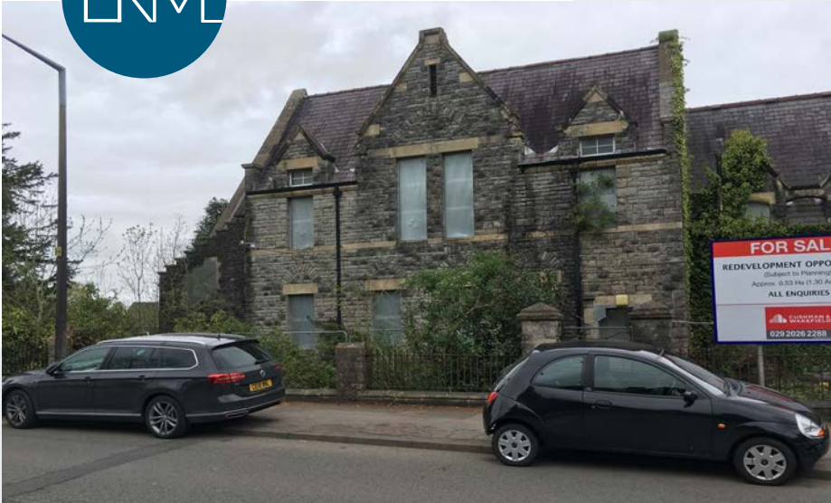
Figure 9 - Part of primary elevation of former school building
