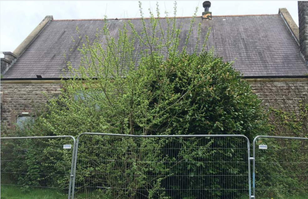
Figure 18 - Side (northern) elevation
