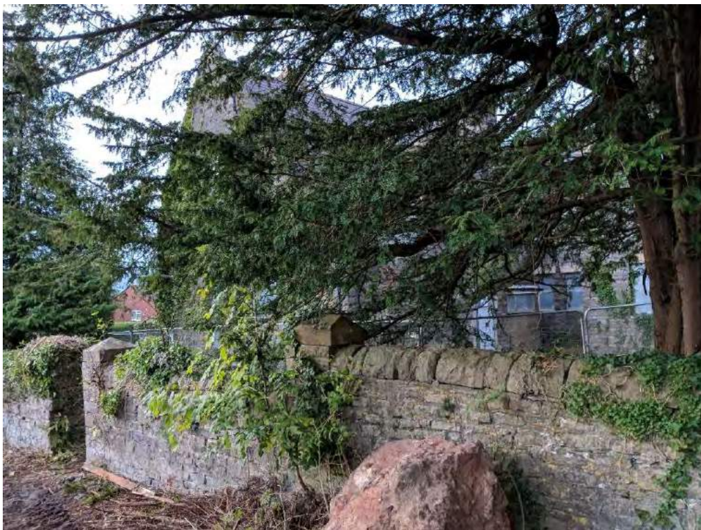
Image EDP 15: The southern extent of the boundary wall.
