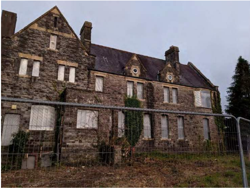
Image EDP 10: North-west facing elevation of the 1896 part of the building.
