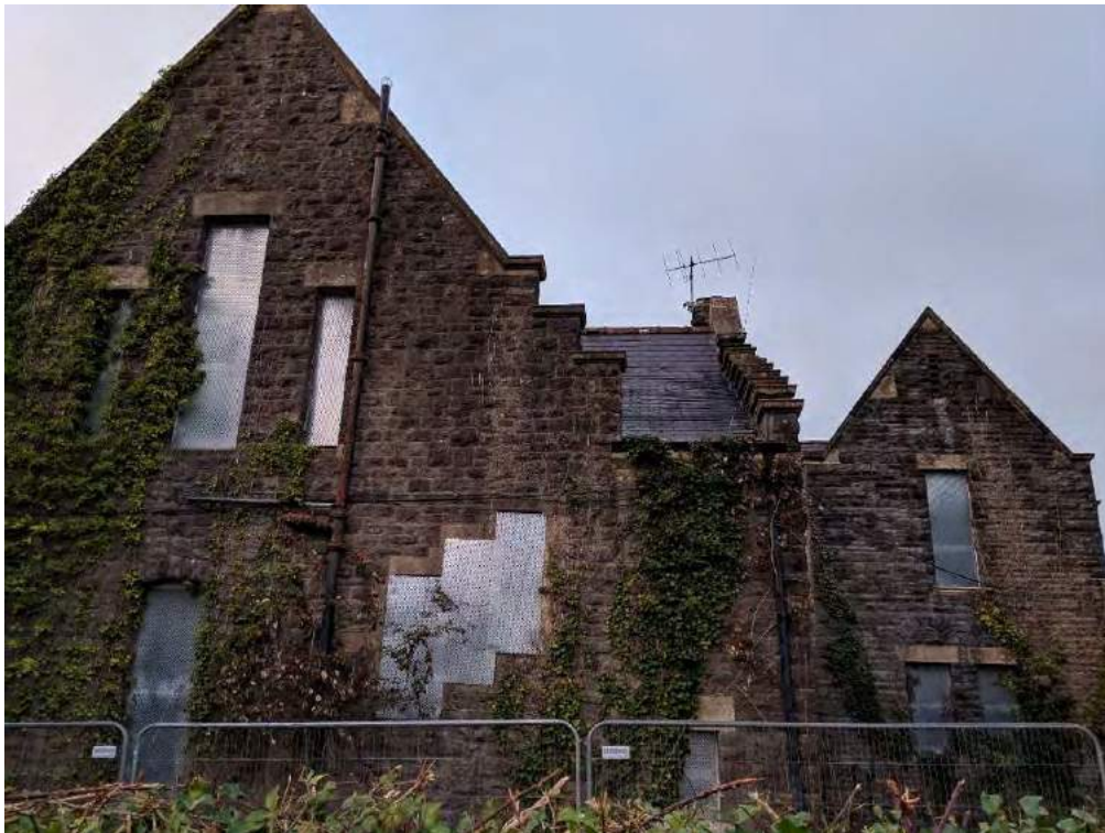
Image EDP 11: South-west facing elevation of the school building.
