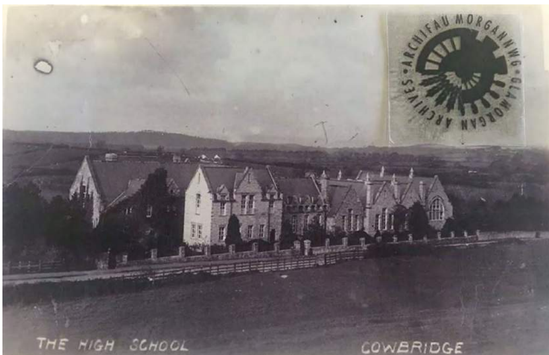
Image EDP 2: Photo of exterior of the school building (1930) (Glamorgan Archives, D1254/3/4).
