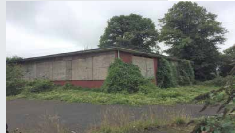
Fig 10 (Above): Existing prefabricated outbuilding ancillary to the main school building
