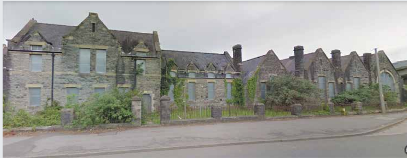
Fig 11 (Above): View of the existing school buildings looking west from Aberthin Road
