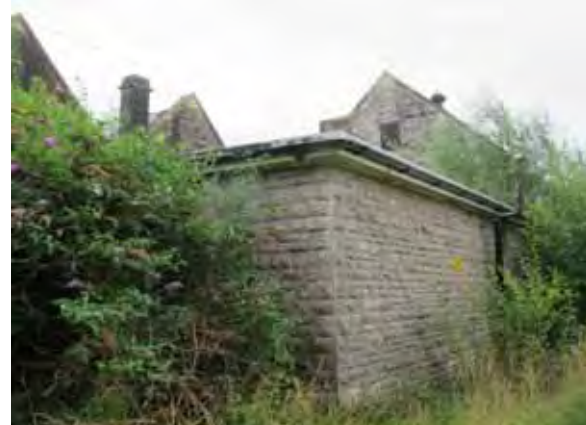
Flat roof room to rear of main school building
