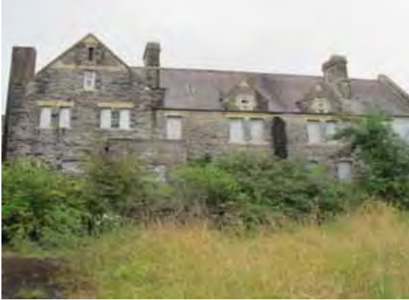
Main school building, north-west aspect
