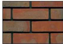
Facing Brickwork
