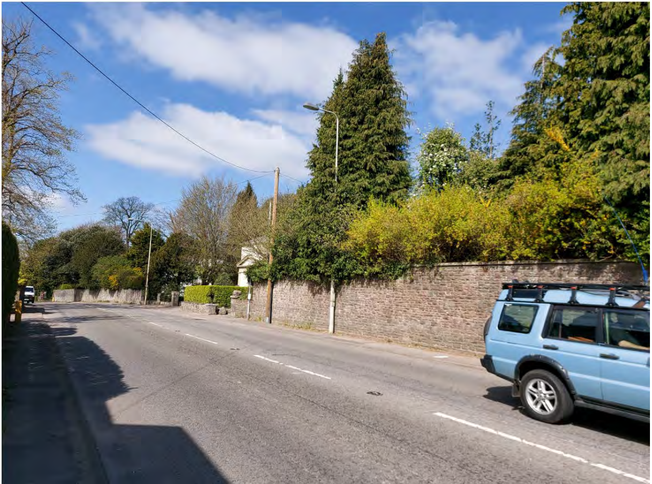
PHOTO OF BOUNDARY WALL
