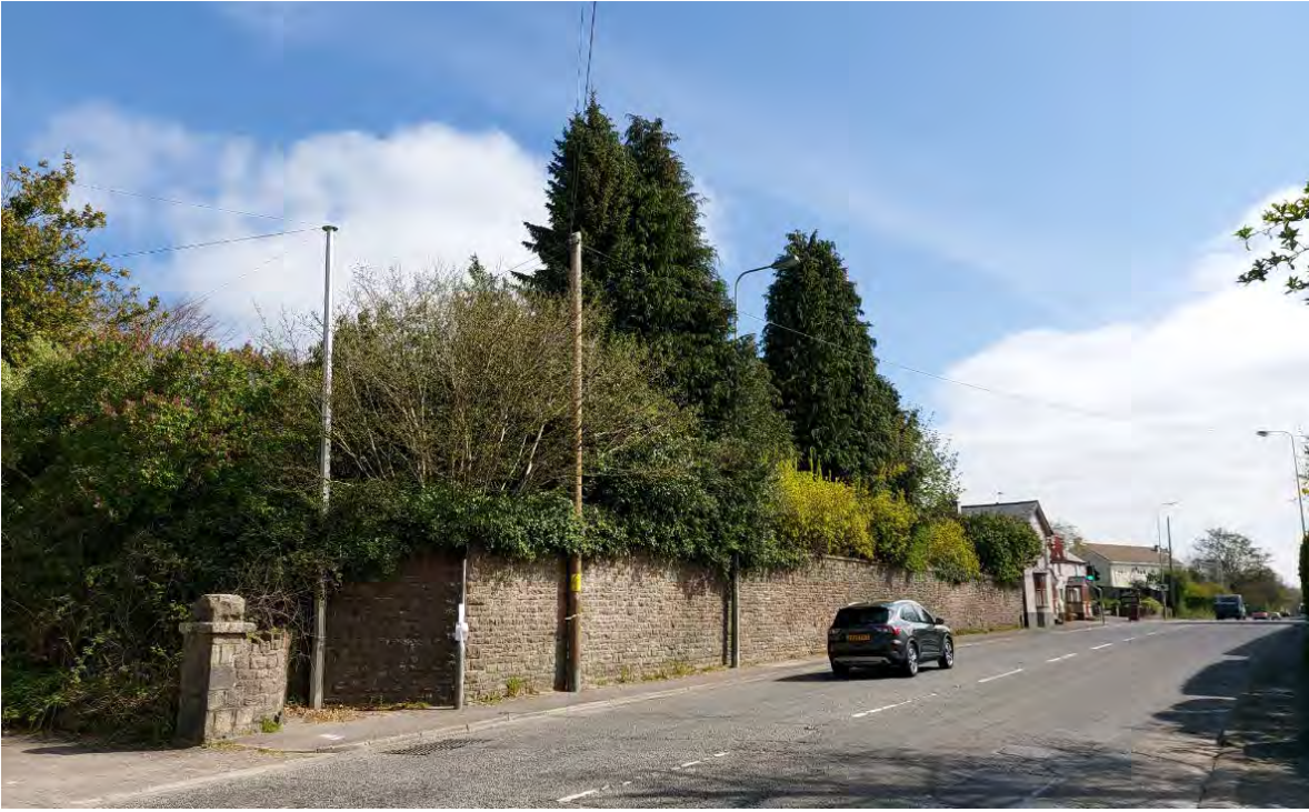
PHOTO OF BOUNDARY WALL
