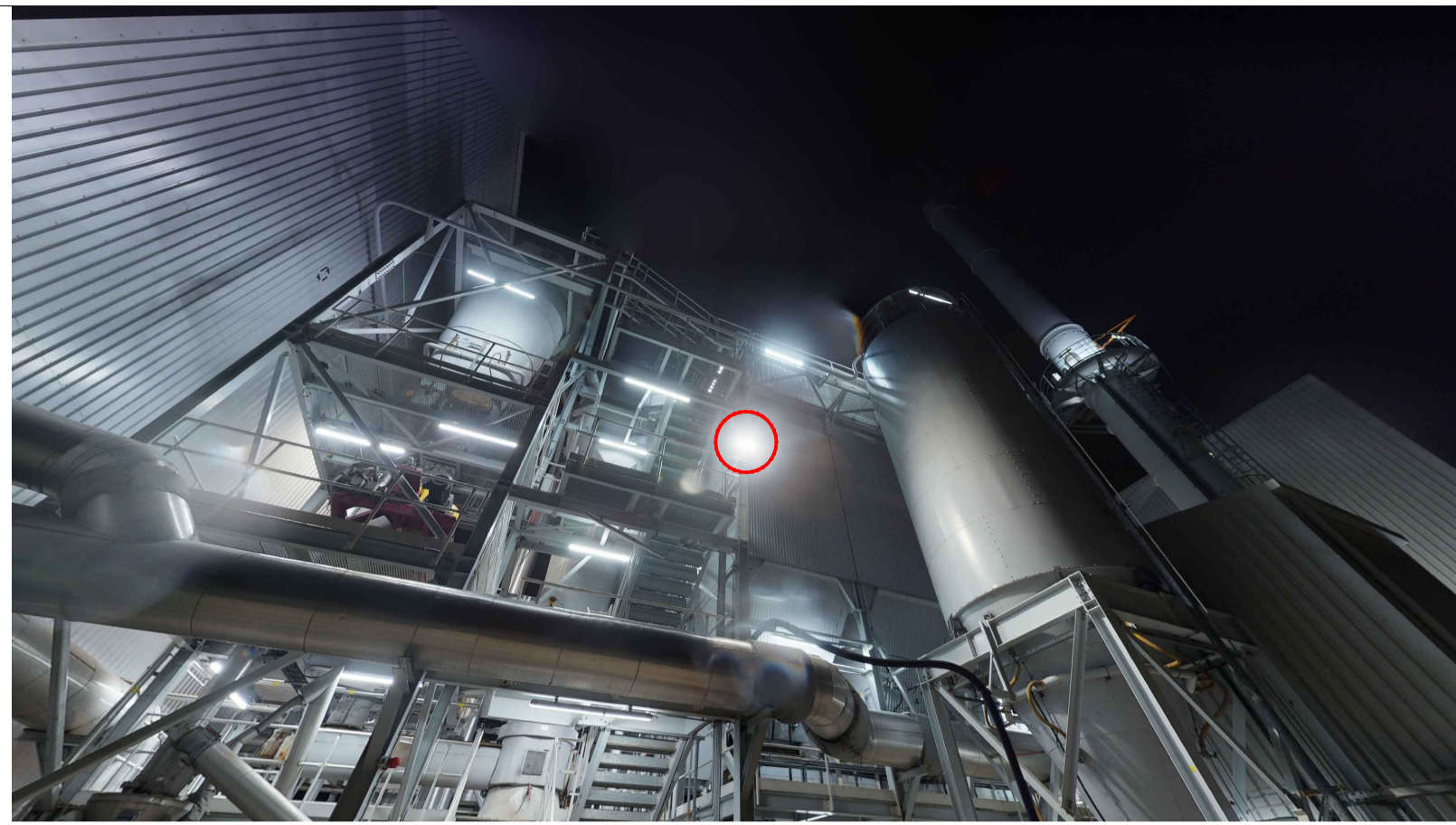
Image 4.1 showing multitude of batten type luminaires and floodlight annotated with red circle
