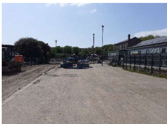
Image EDP 3.9: View of the Site looking east with railway siding/Barry Goodsheds on the right.
