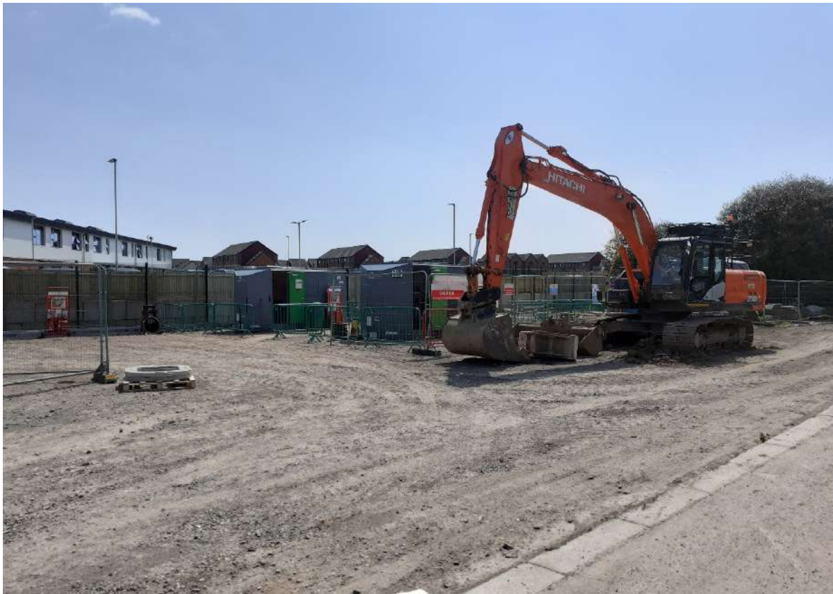
Image EDP 3.11: Site compound for adjacent construction works.
