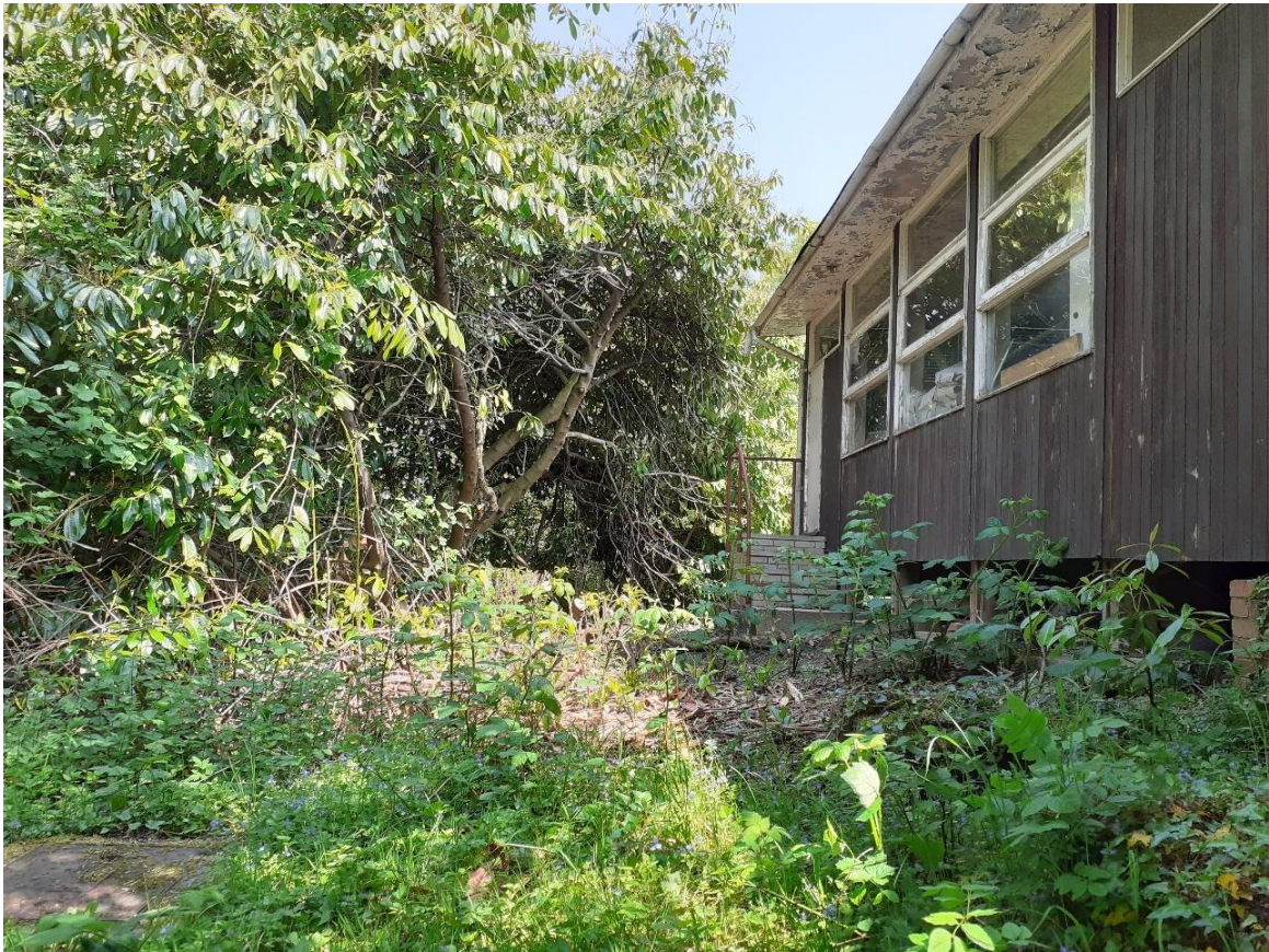
Image EDP A2.7: Cherry laurel between buildings B3 and B4 .
