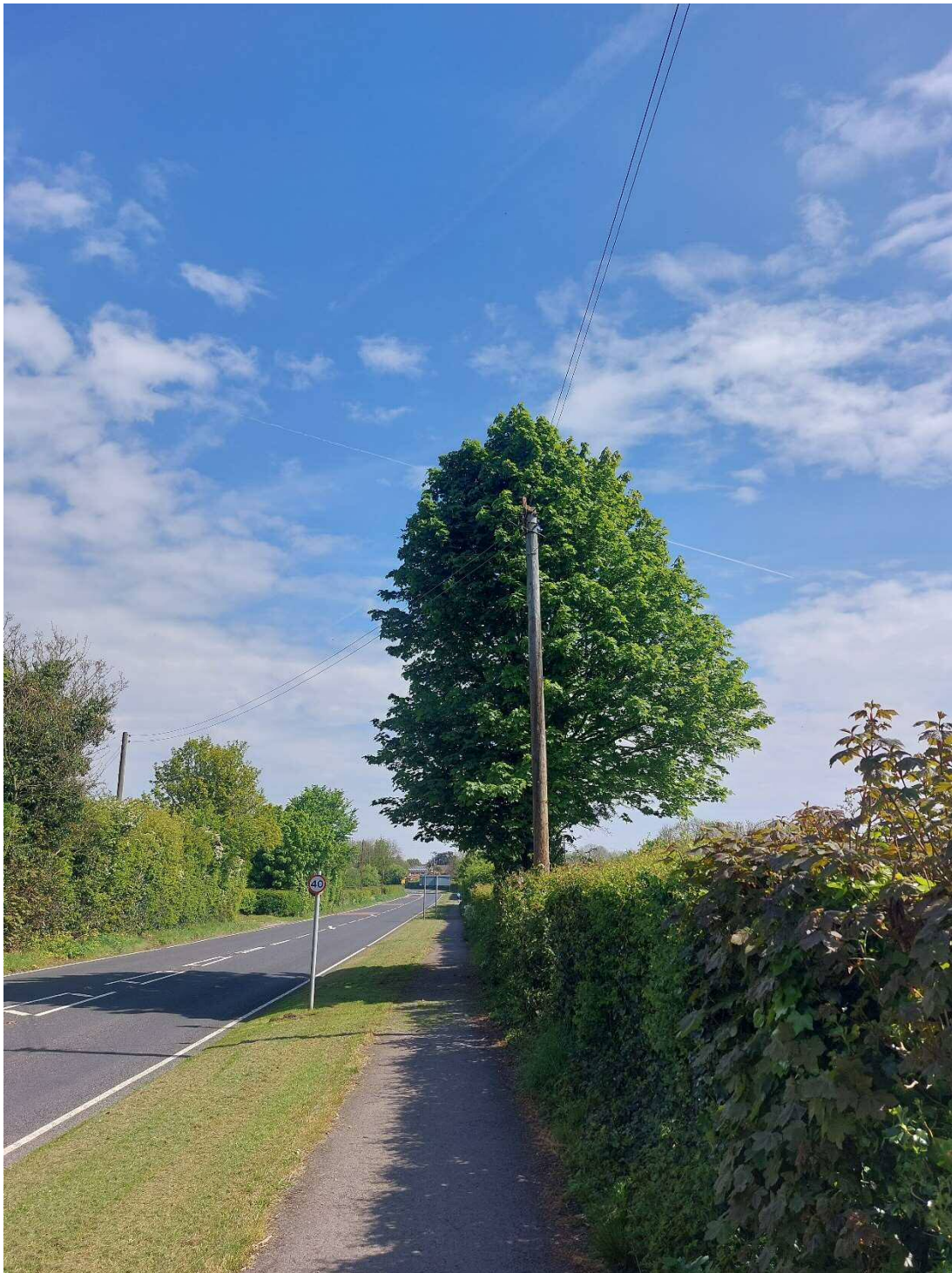
Photograph 5. Tree 5 - Roadside tree of reasonable form. Provides limited screening from the road. Tree growing out of hedgerow. Crown within 2-m of low voltage overhead powerlines.
