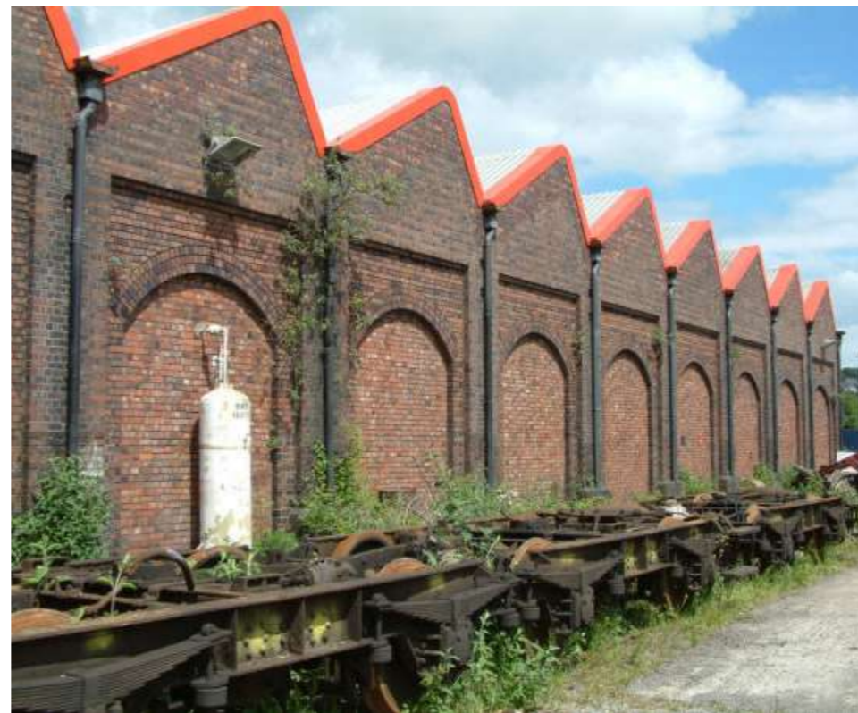
Railway shed, Barry Station
