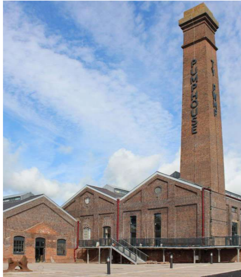
Pumphouse, Barry Innovation Quarter
