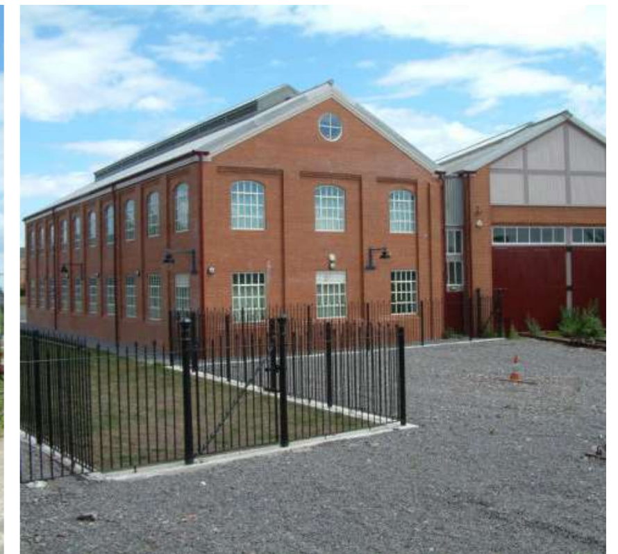
Former railway sheds, Barry Innovation Quarter
