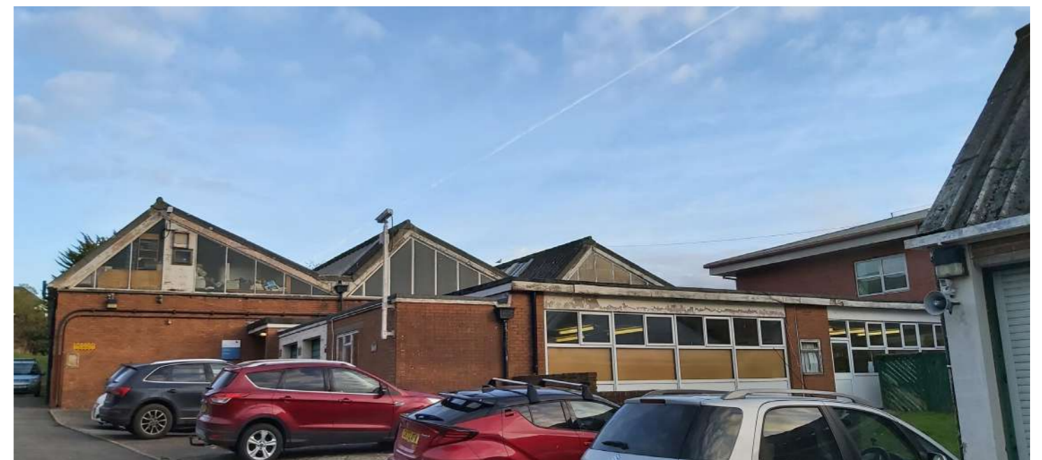
Photographs of the existing Barry Campus on Colcot Road
