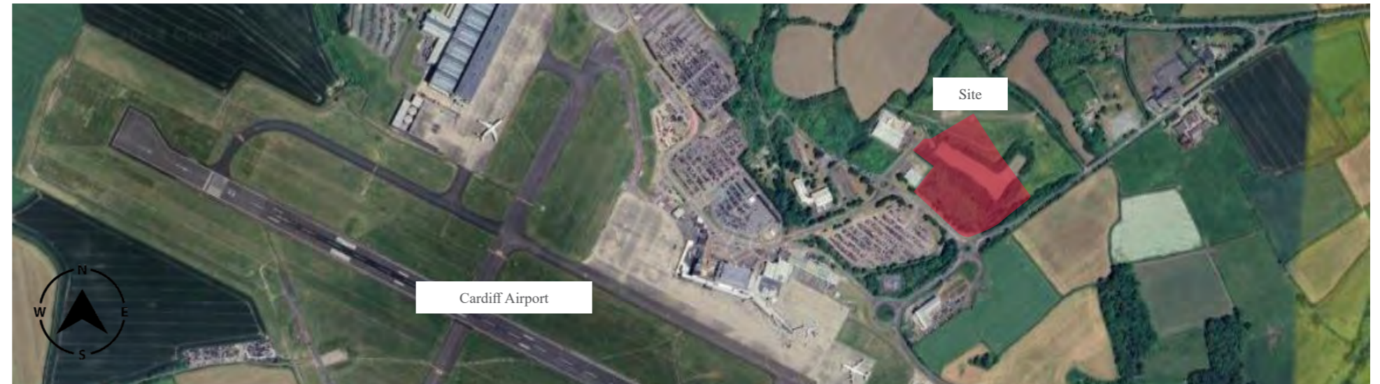
Figure 2: Site location with the proposed site highlighted in red.
