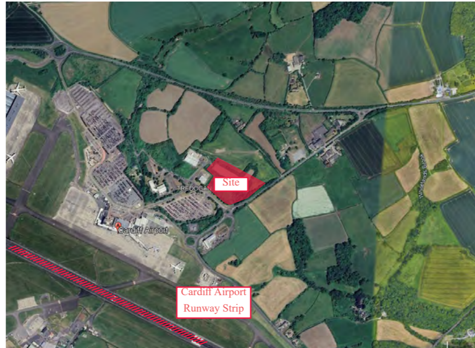
Figure 32: CAVC, ATC - Surrounding site context. Source: Google Earth
