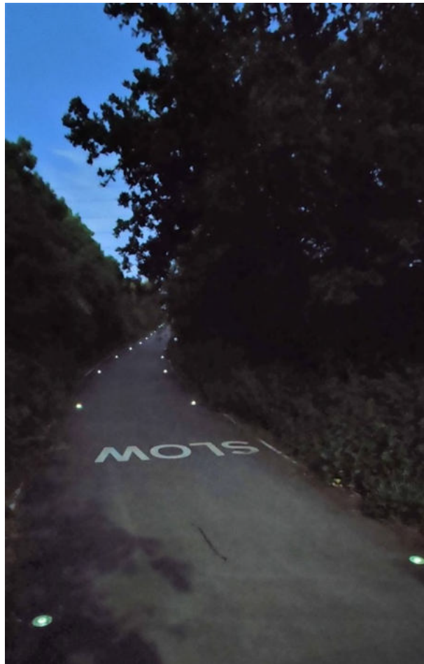
Photo 4: Waymarkers installed on a multi-user path in Worcester. Image credit: Cody Levine.
