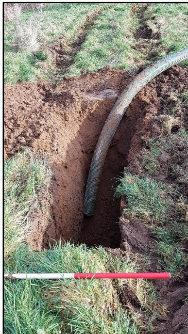
Plate 8. Test pit number 5A. Looking east. Scale 1m with 0.5m division.
