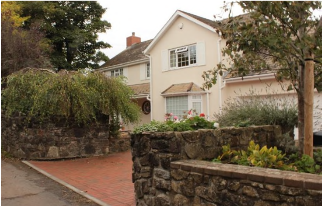
Figure 15 Modern development with rendered elevations. The brick paving to the driveway is at odds with the character and appearance of the conservation area, introducing a suburban character.
