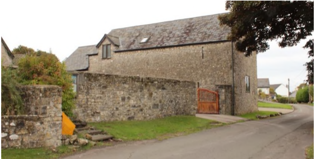
Figure 10 A converted barn to the west of Great House, Church Street.
