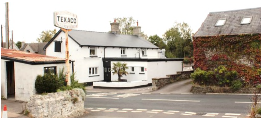
Figure 12 The Carne Arms and barn on the B4268 from Church Street.
