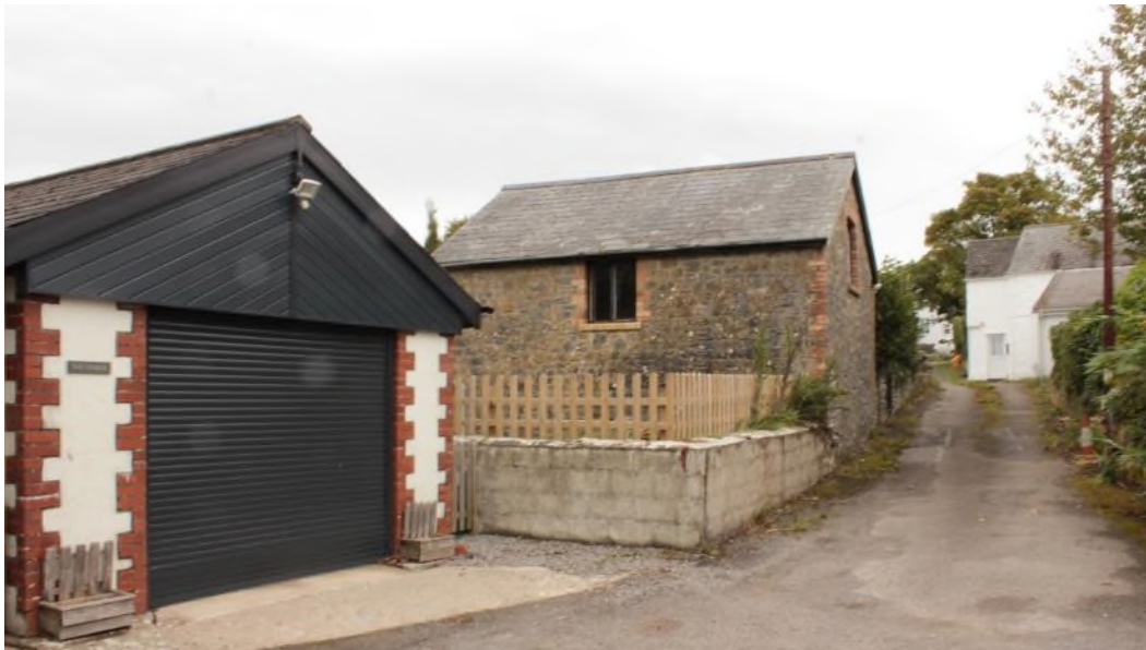
Figure 11 A small converted former agricultural building on Squire Street.
