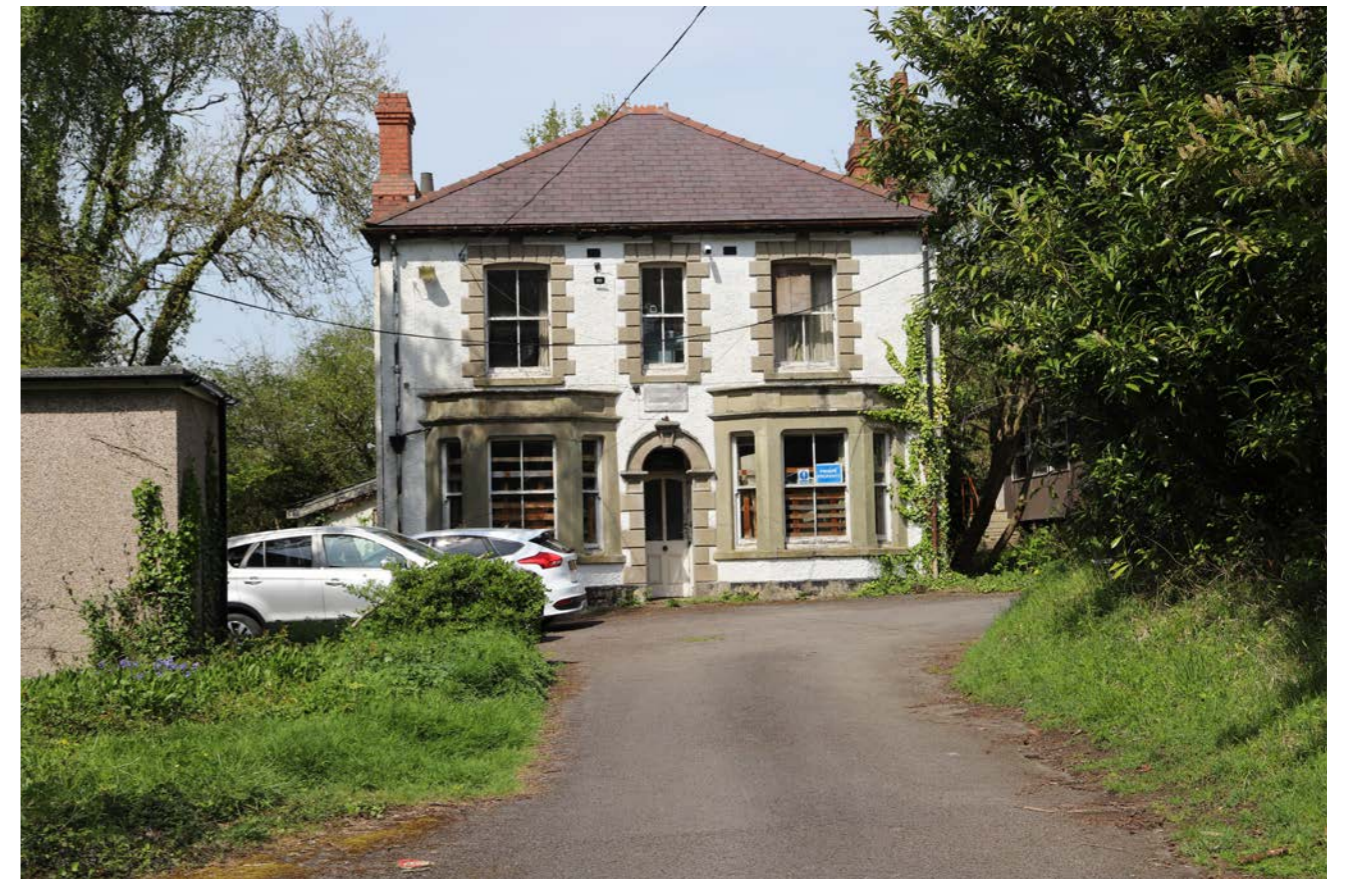
Figure 2.2: Existing building to be retained and renovated for residential use
