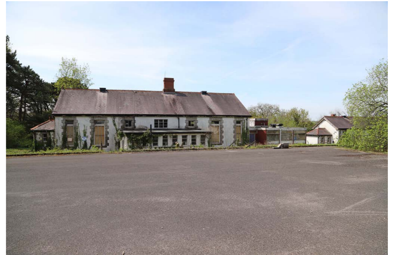
Figure 1.2: Existing vacant buildings on site
