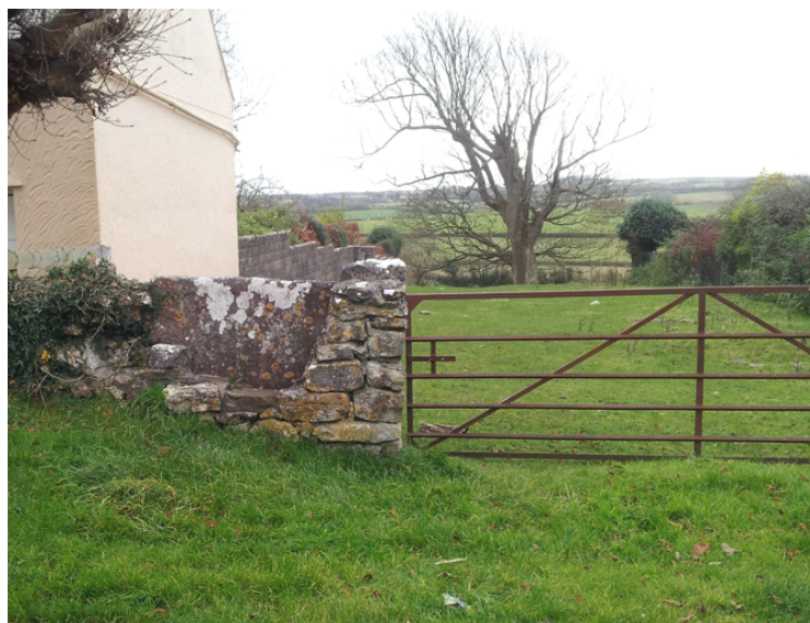
Stile before it was removed.
