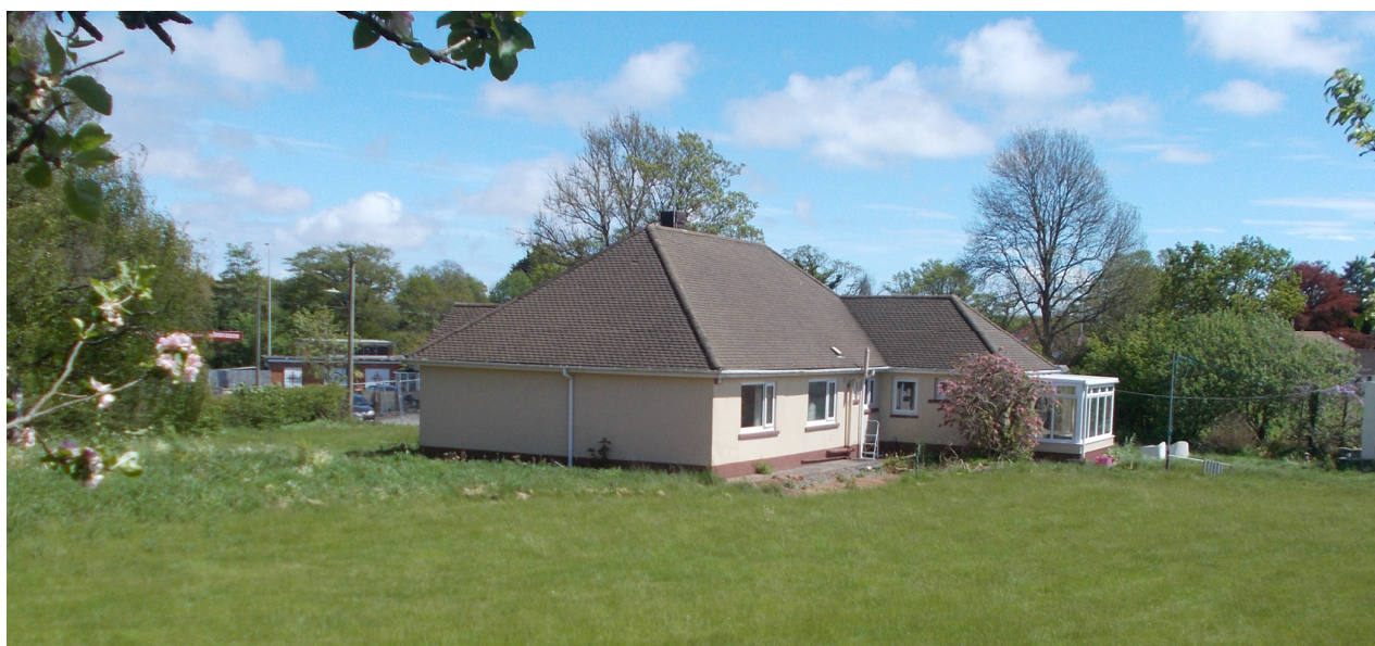
View of side/rear of existing dwelling eastwards
