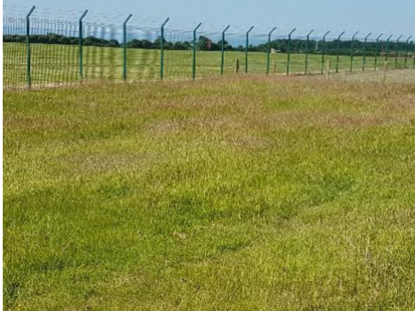
Bro Tathan West and Airfield Fence
