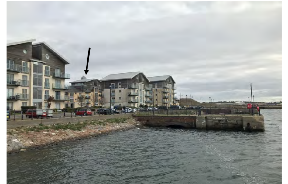
Figure 40: View north east from projecting platform into Dock no.1 from Y Rhodfa.
