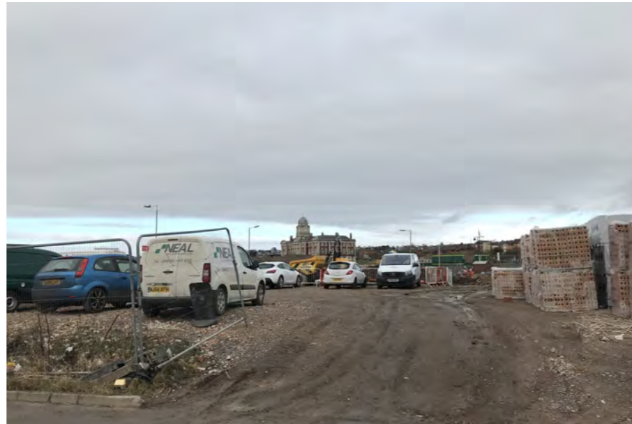
Figure 42: View north west from a position north of David Davies Road and a short distance west of the 20th century commercial units on Woodham Road.
