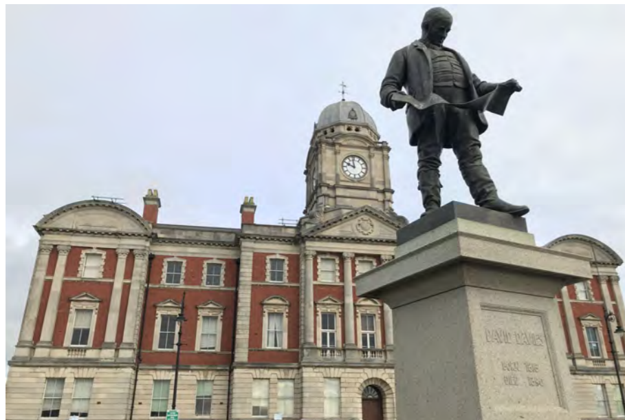
Figure 35: Close view of David Davies Statue and principal (south) elevation of the Former Docks Office
