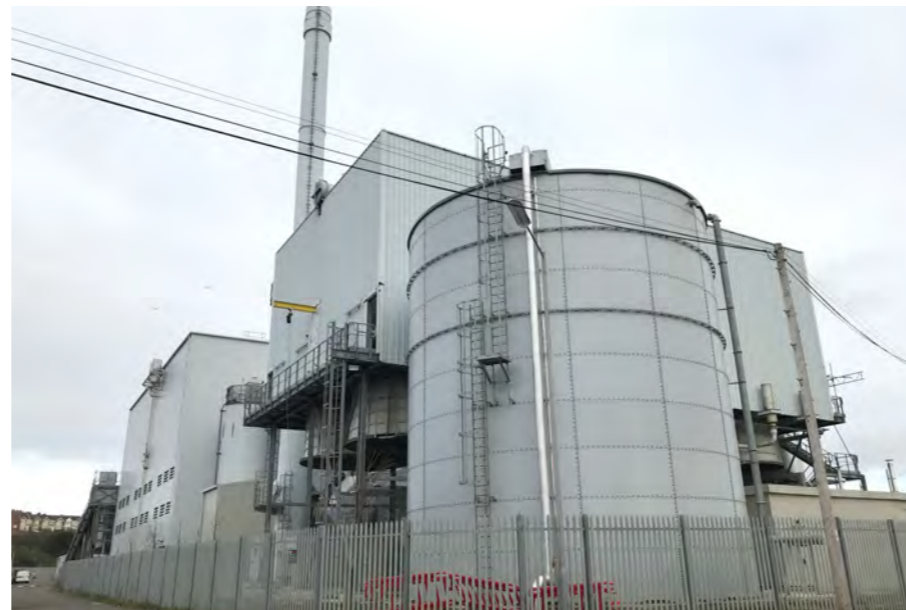
Figure 24: General view of Biomass Facility from the south on David Davies Road.
