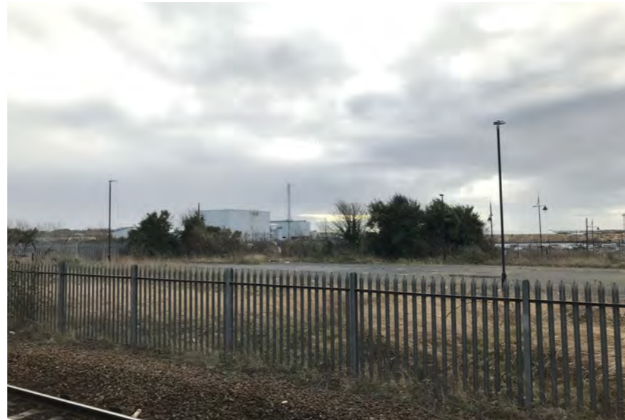
Figure 16: View to Site, looking approximately south east from south platform at Barry Docks train station.
