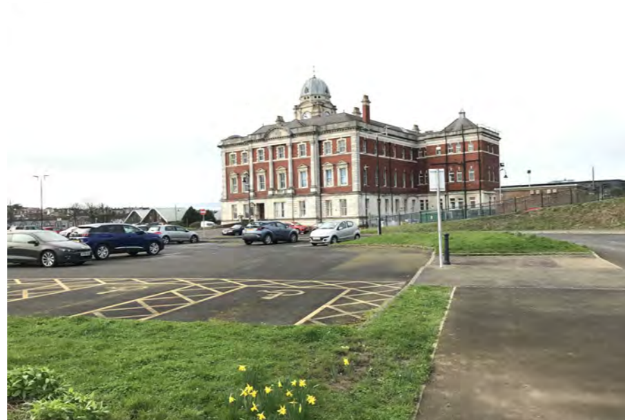
Figure 33: View to Former Docks Office and lampposts on eastern side across car park looking approximately south west
