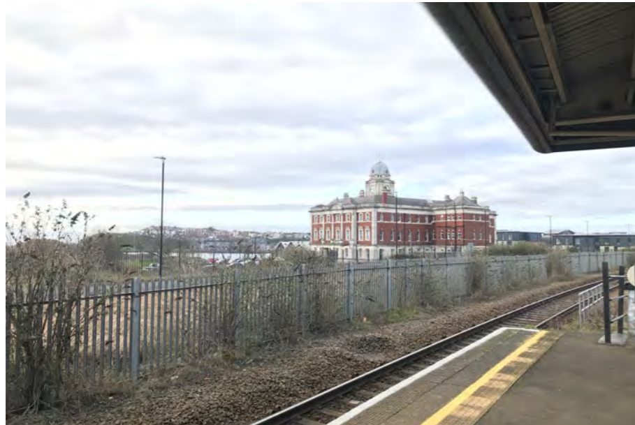
Figure 32: View south west to Former Docks Offices.
