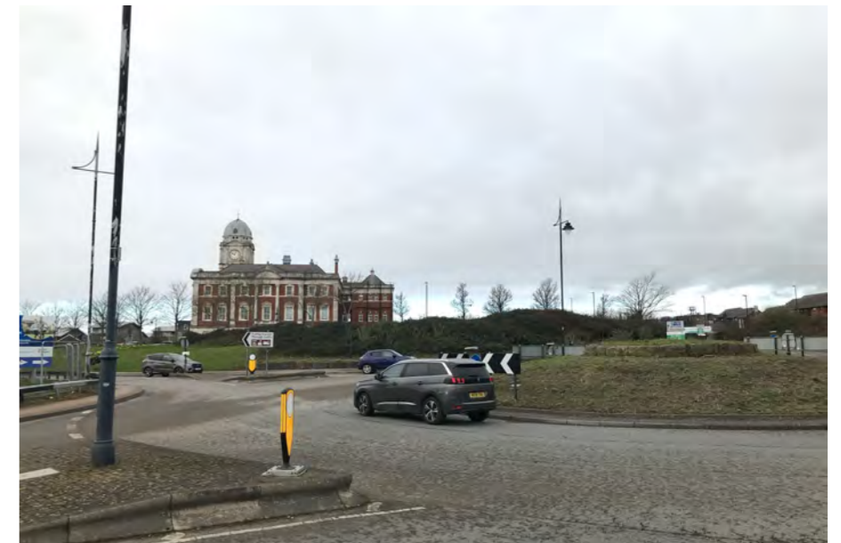
Figure 37: General view west over the Ffordd Y Mileniwm roundabout. Traffic noise and visual impacts are a notable element in the character of the immediate setting of the group of assets at the Former Docks Office.
