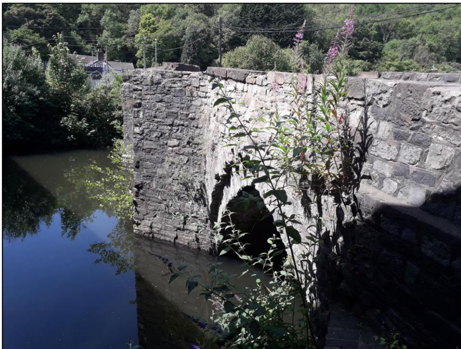
Plate 7. View of Leckwith Bridge 00134s/GM014/LB13748/LB26487/24126 from 307689 towards the north
