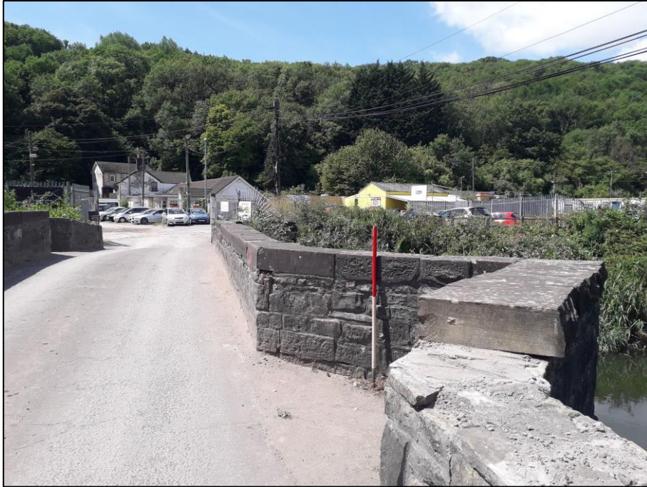
Plate 6. Eastern end of Leckwith Bridge 00134s/GM014/LB13748/LB26487/24126 (Scale: 0.5m divisions)
