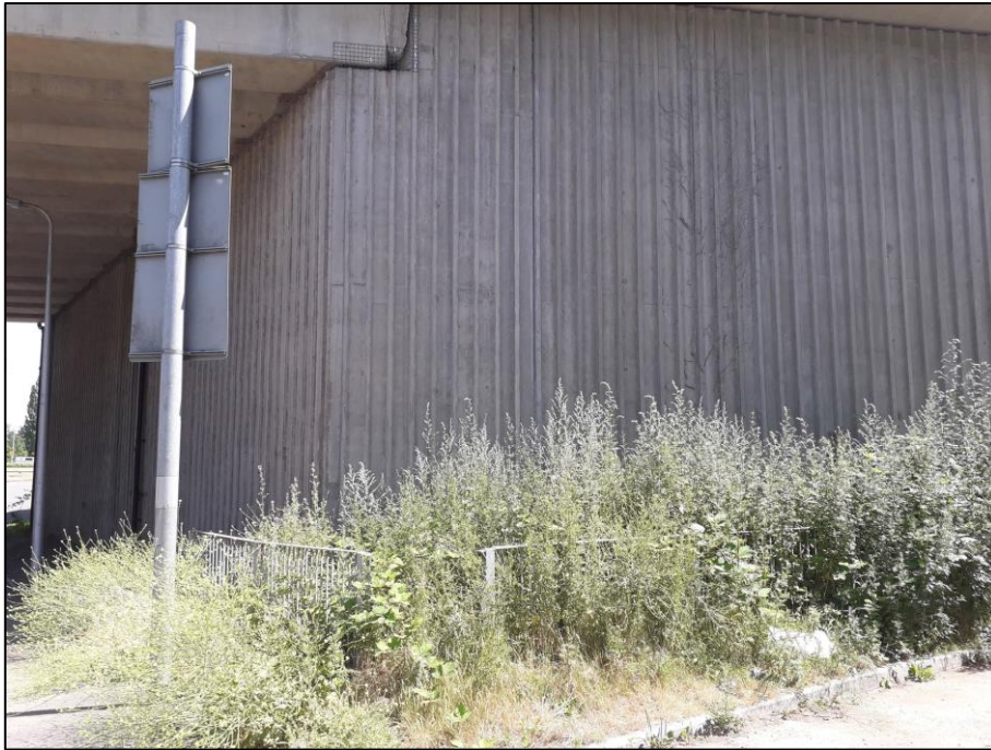
Plate 16. Former location of cottage LQ003, view to the east
