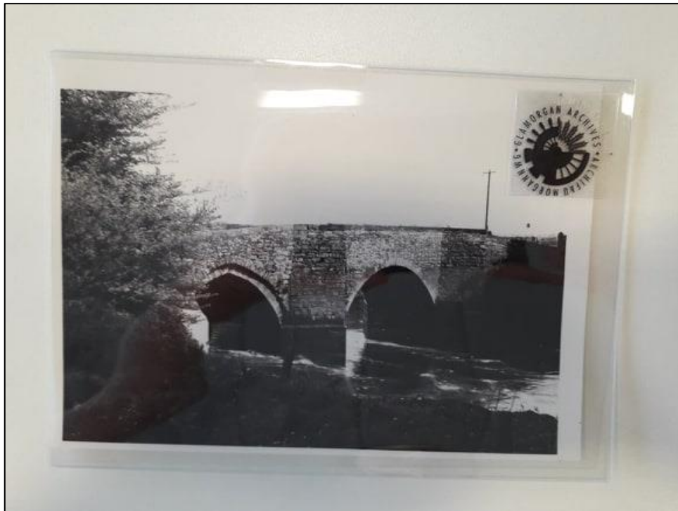
Plate 3. Photograph of Leckwith Bridge (00134S/GM014/LB13748/LB26487/24126) to the west (1952-1973)
