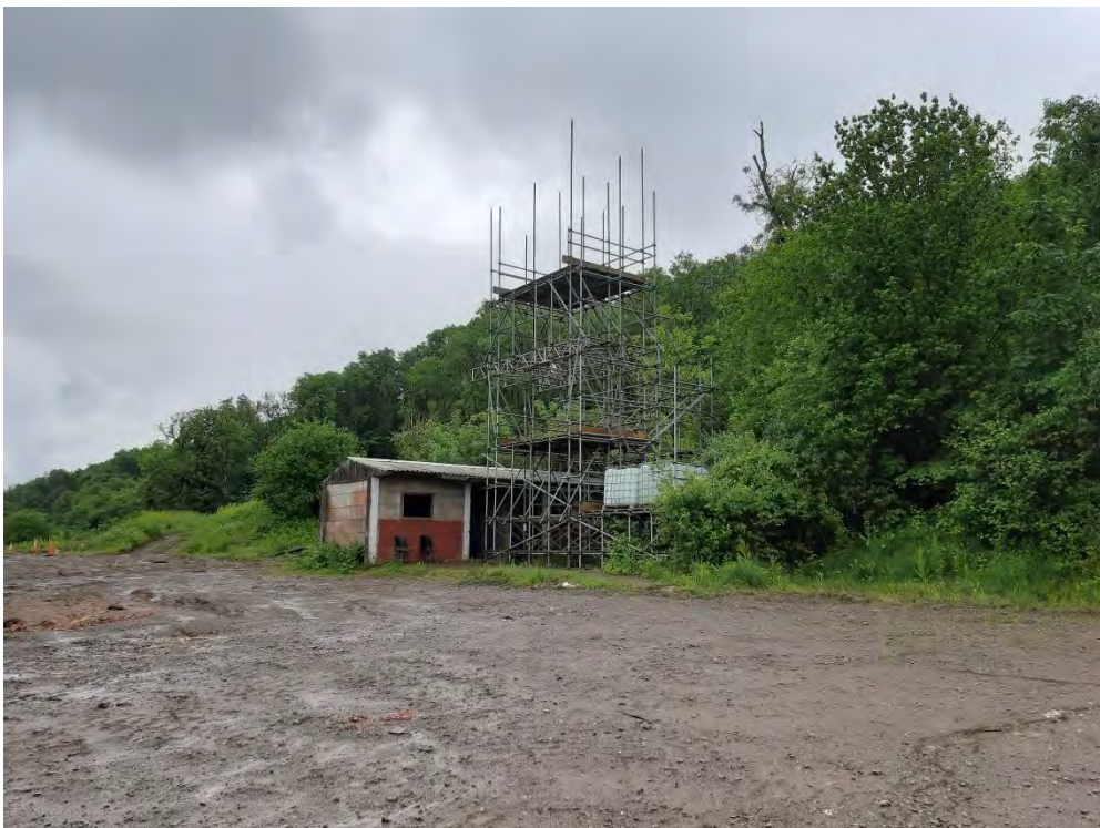
Photograph R - Crane platform used for crane and digger operator training in the south of the site (WSP, June 2019)
