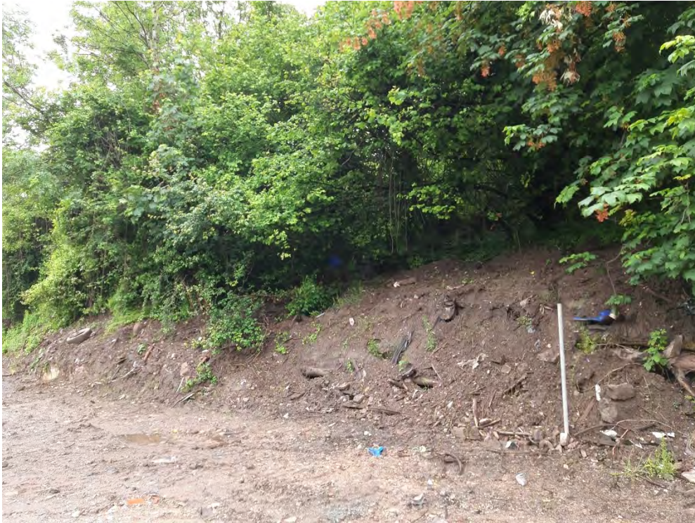
Photograph O - Made Ground embankment along the western site boundary in the south of the site (WSP, June 2019)
