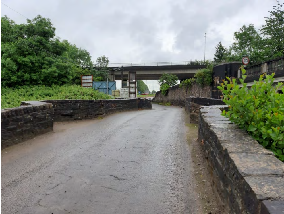
Photograph A - The narrow road bridge forming the only site access (WSP, June 2019)
