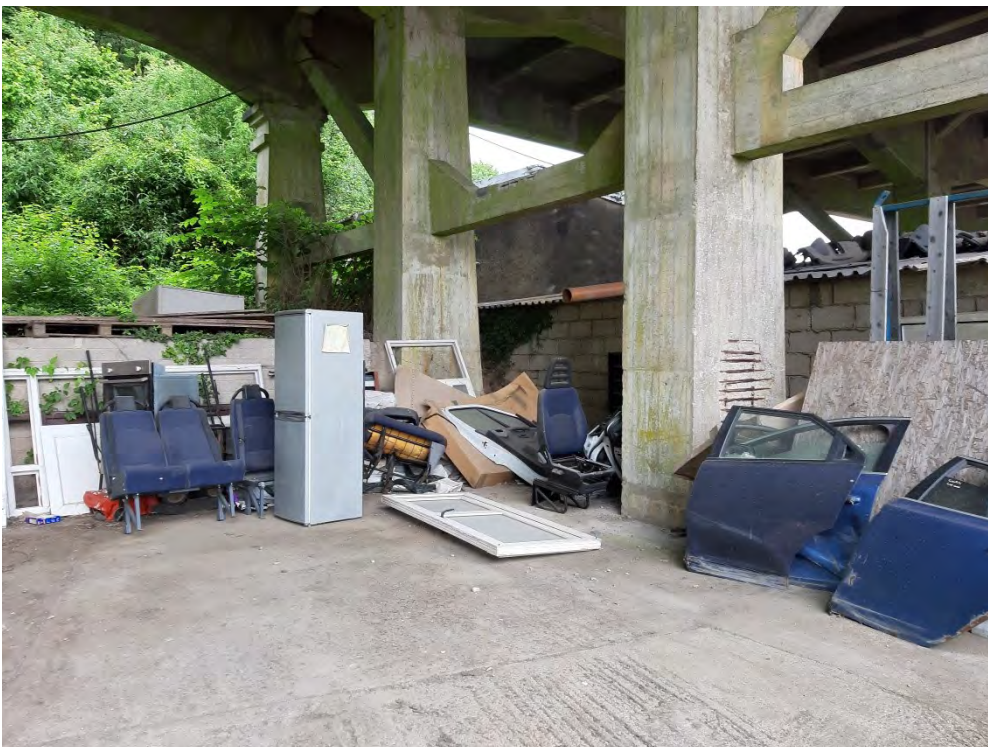
Photograph L - Extensive fly tipping around the centre of the site (WSP, June 2019)
