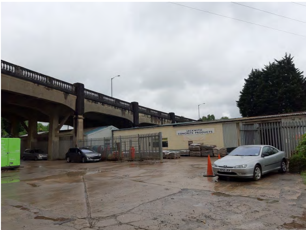
Photograph J - Concrete works in the centre of the site (WSP, June 2019)
