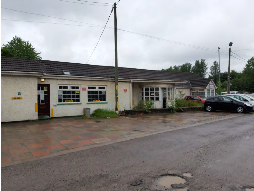
Photograph I - Office premises in the centre of the site (WSP, June 2019)
