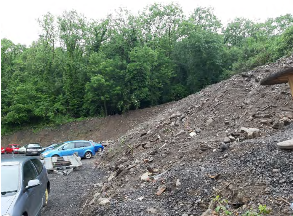
Photograph D - Large embankment along the northern boundary of the site comprising historical landfill waste (WSP, June 2019)
