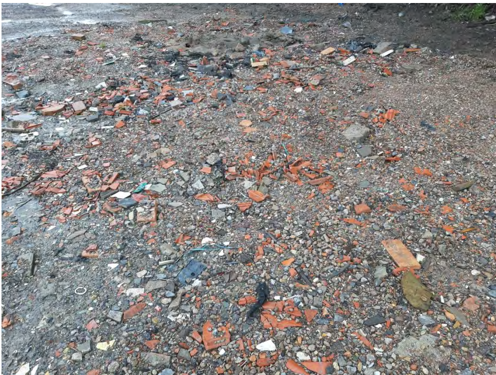
Photograph N - Made Ground cover in the south of the site (WSP, June 2019)
