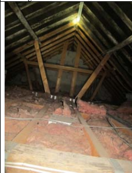
Building 1 loft void interior
