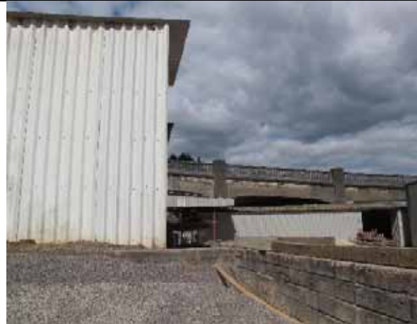
Building 6 and viaduct
