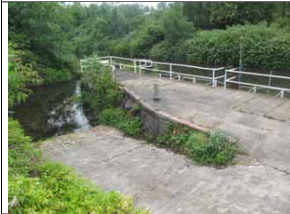
Jetty to the east of the site
