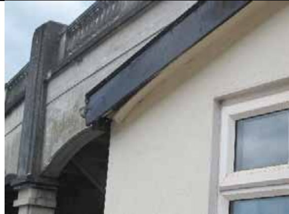
Building 6 – external features
