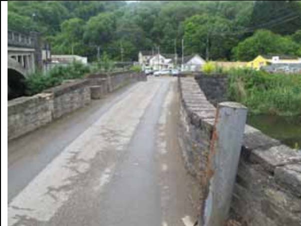
Road bridge crossing the Ely to enter the site
