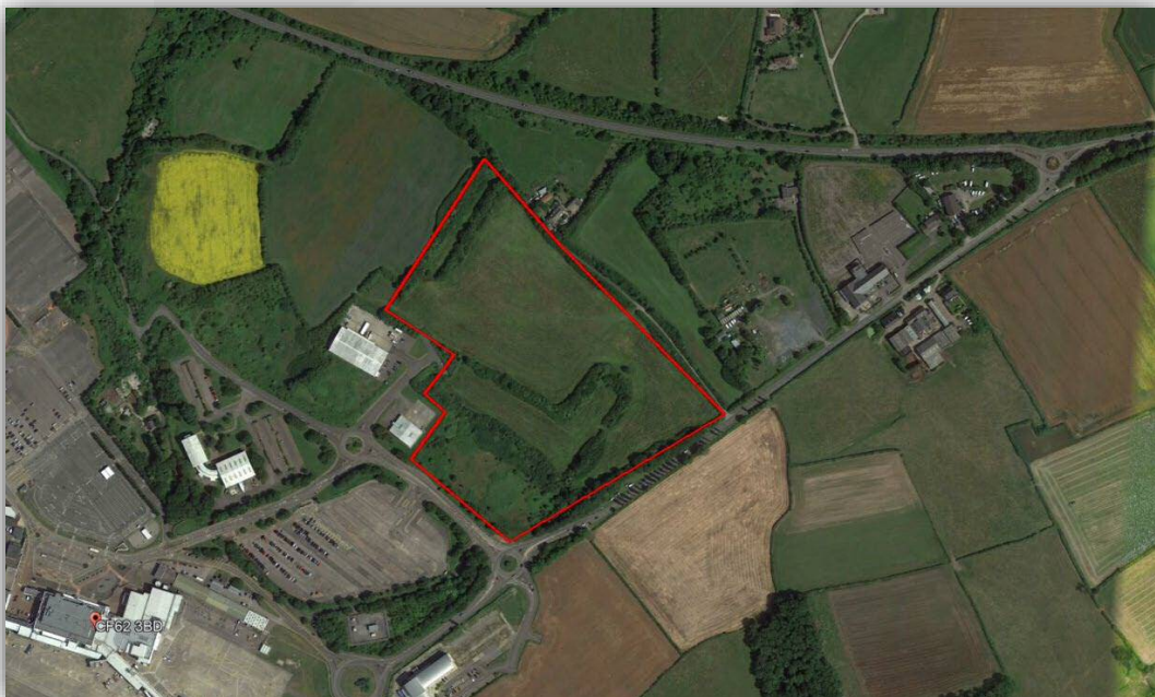
Figure 1: Aerial Image of site with approximate red line boundary area surveyed (Google Earth)
